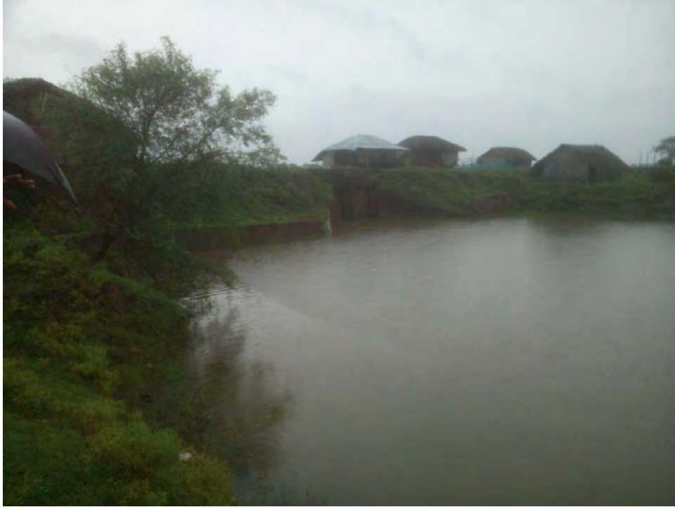
Polder 17/2, Closed regulator near 4-vent Existing regulator
