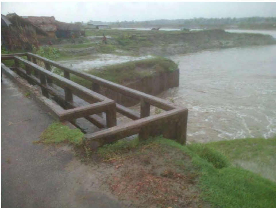
Polder 17/2, Existing 4-vent regulator
