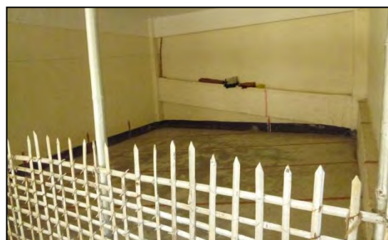
Photo 4.26: MPCS's Ground Floor in Chakamaiya Union Used as Prayer Room ( Source: Field Visit, February 2013)
