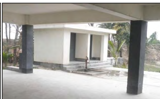
Photo 3.7: Tube-well and Toilet is in Ground floor of MPCS in Dhankhali Union
