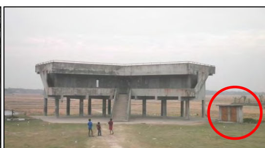
Photo-5.4: MPCSS constructed by CARITAS Mithaganj Union which toilets are outside the main building
