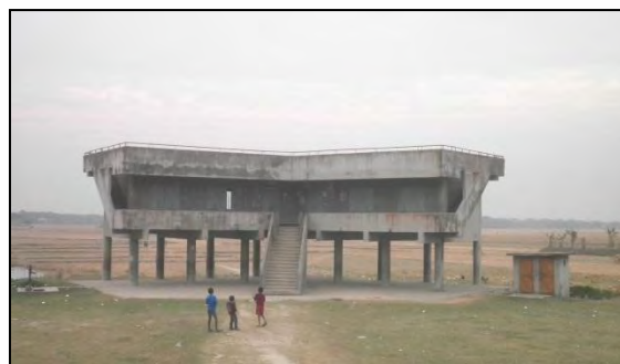
Photo 5.16: No boundary wall of MPCSS in Mithaganj Union made by CARITAS (Source: Field Visit, February 2013)
