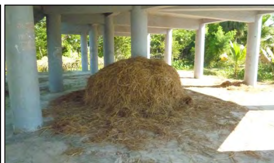
Photo 4.16: MPCSS in Latachapali Union used as Store Room for Crops
