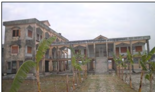
Photo3.12: L- shape Union Parishad cum Cyclone Shelter in Lalua Union
