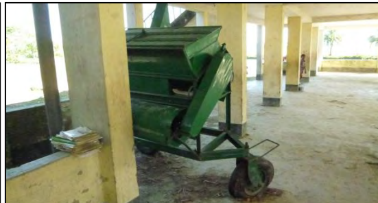
Photo 4.7: MPCs in Lalua Union used as Garage
