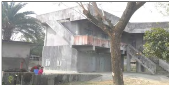
Photo 4.8: MPCs in Tiakhali Union used as Residence by Local People
