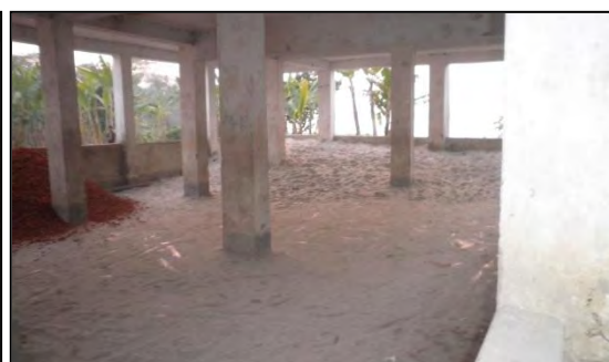
Photo 4.18: MPCSS in Lalua Union used as to keep Construction Materials
