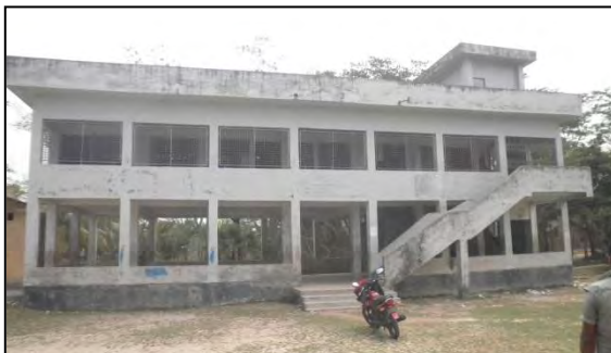
Photo3.11: Rectangular shape School cum Cyclone Shelter in Chakamaiya Union
