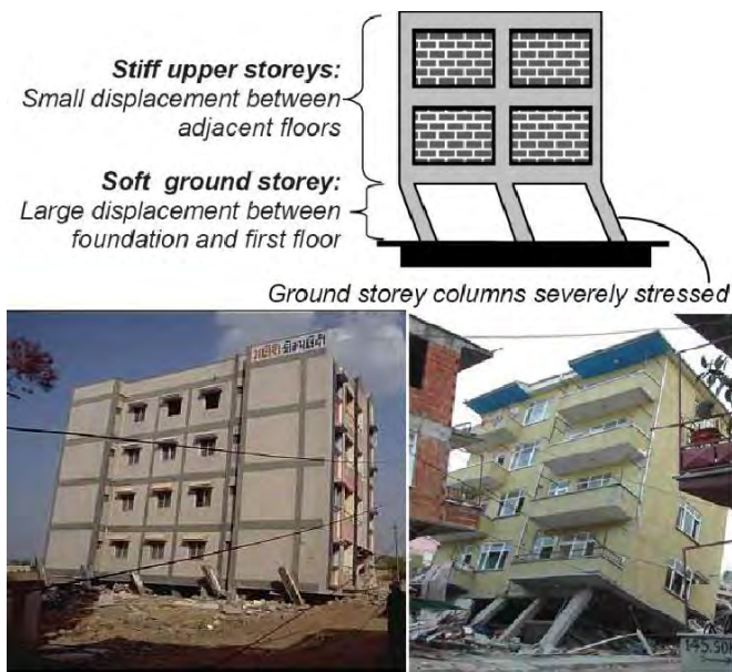
Figure 1.3: Failure due to large lateral displacement in soft storey
