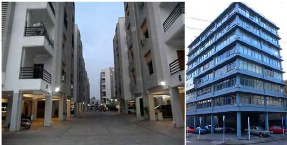
Figure 1.1: Soft storey reinforced concrete buildings
