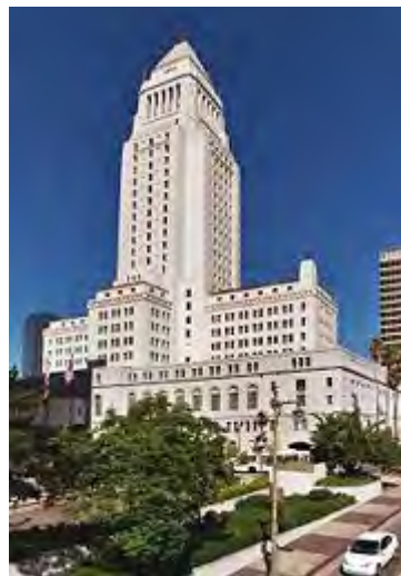
Figure 2.5: Base-isolated LA City Hall
