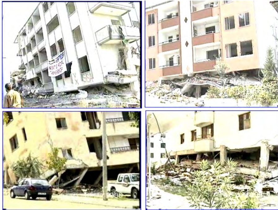
Figure 3.4: Damage to soft storey of Izmit Earthquake (Yalova-Gölcük)
