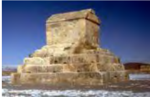
Figure 2.4: Mausoleum of Cyrus, the oldest base-isolated structure in the world
