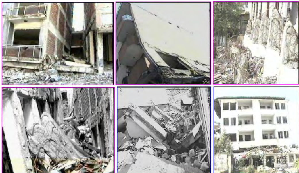
Figure 3.3: Damage of Izmit earthquake (Adapazarı)
