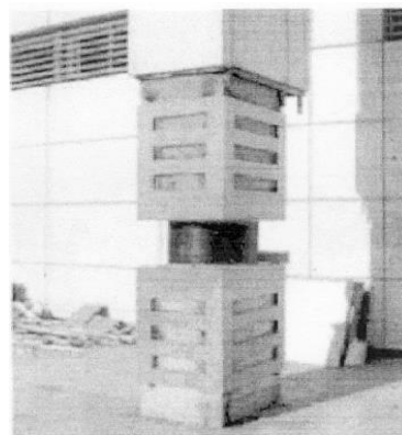
Figure 2.32 Steel Jackets replacing severed reinforcing bars
