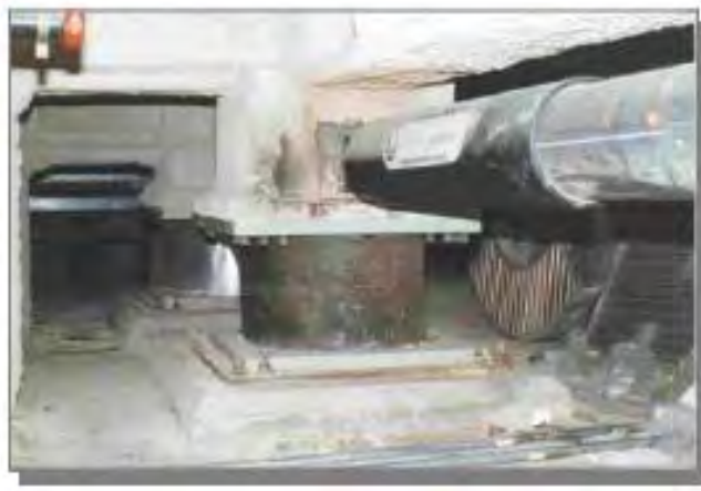
Figure 2.27: Isolator Installation in Building
