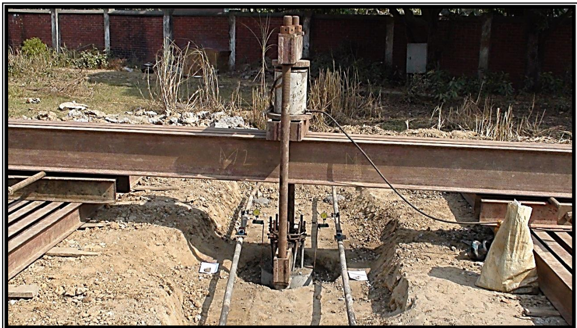
Figure 3.5: Photograph showing test set-up for uplift test at Baridhara site (S-01)
