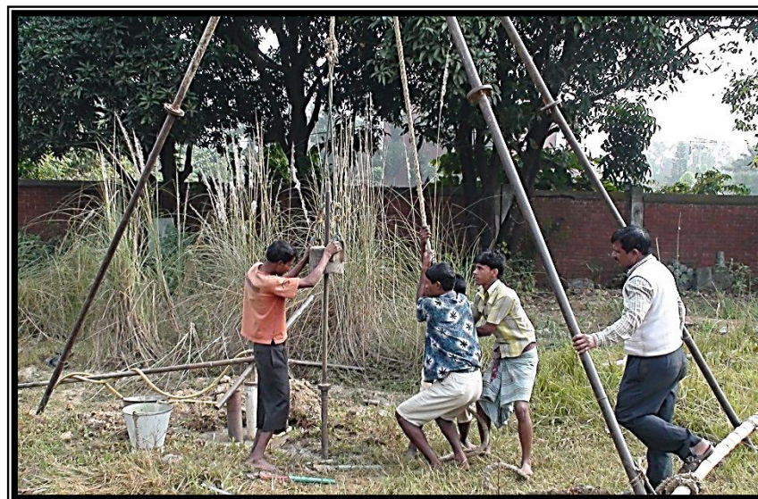
Figure 3.3: Photograph showing sub-soil investigation at Baridhara site (S-01)
