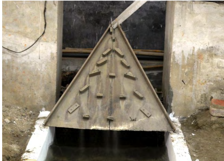
Figure 5.21: Wooden structure for sediment distribution
