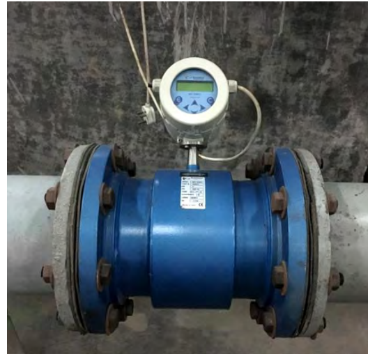
Figure 5.15: Electromagnetic flow meter
