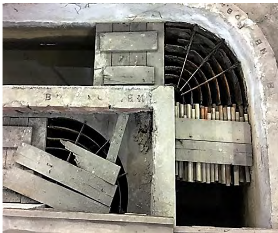
Figure 5.12: Guiding vanes and tubes
