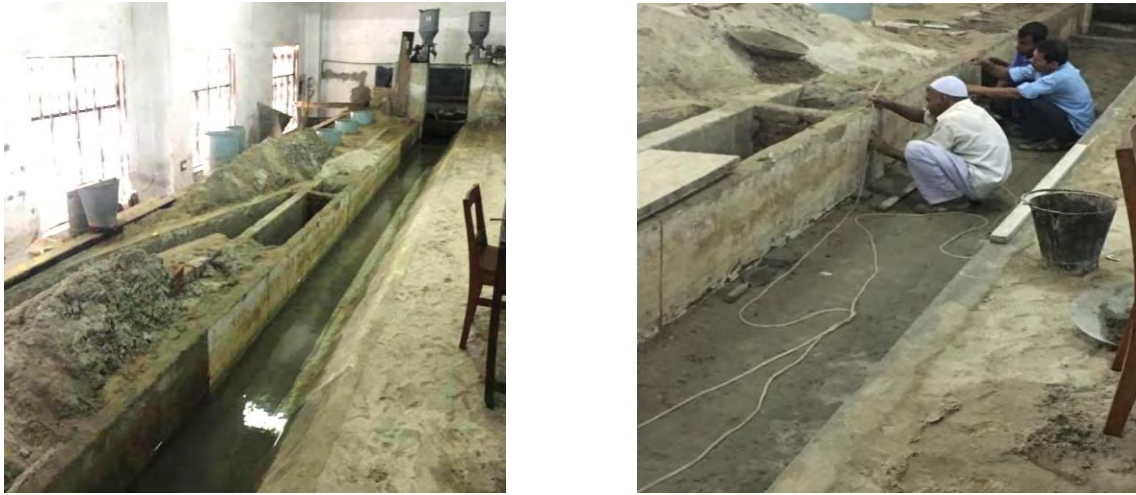
Figure 5.1: Experimental channel before reconstruction (left), during reconstruction (right)
