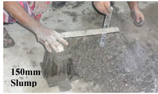
(b) Slump for column mid zone concrete
