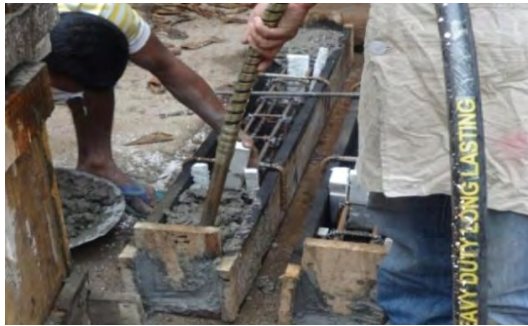
(c) Compacting of concrete
