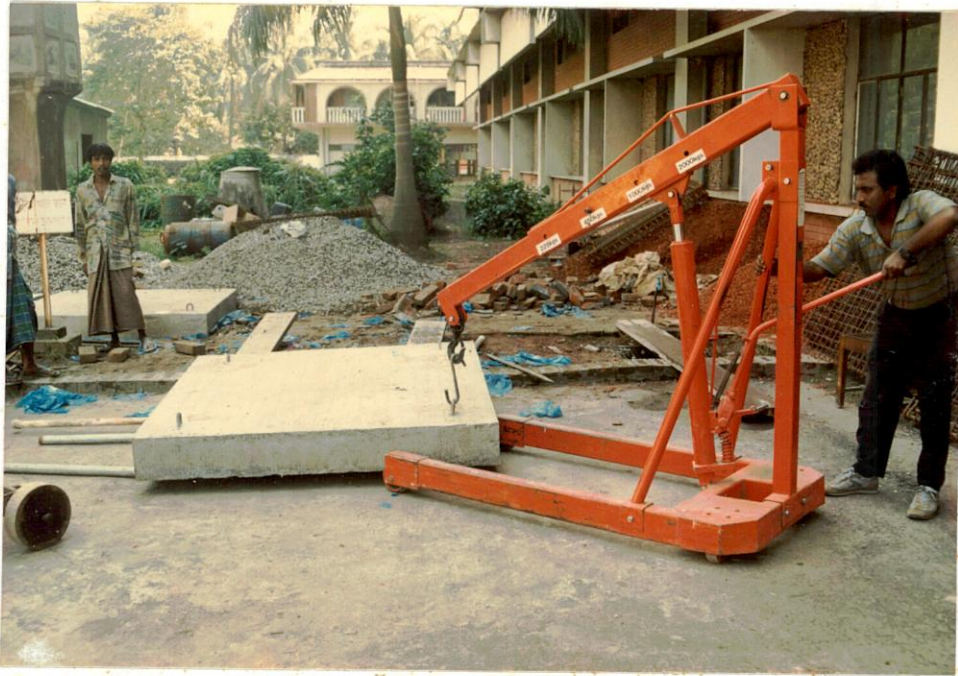
Figure C-1 Lifting of the slab at the casting yard.
