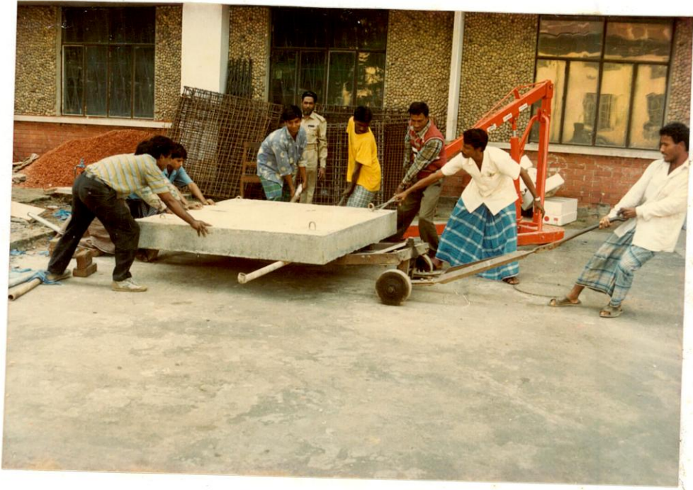
Figure C-3 Trolley along with slab being pushed and pulled towards the laboratory.
