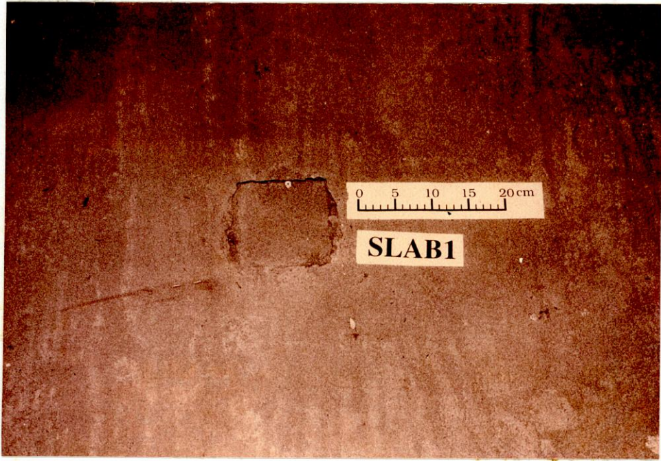
Figure 4.2 Typical cracking pattern on the top surface of a model slab
