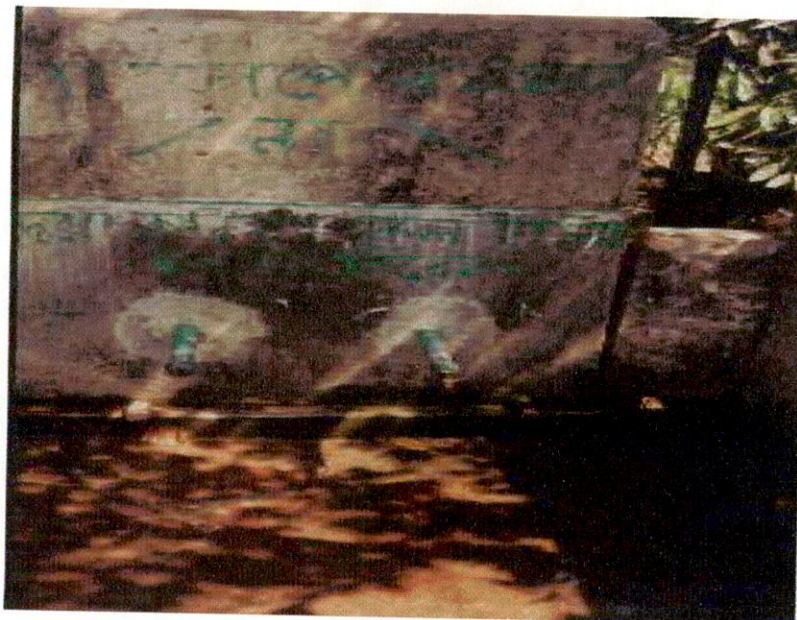
Plate-4.5: Stick has been used instead of Tap to control Flow at Shyamnagar, Satkhira
