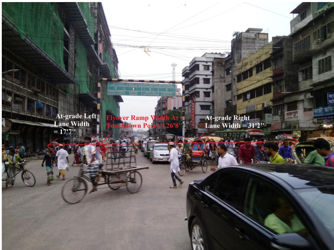
Figure 4.37: At-Grade Lane Width Reduction at the Touchdown Point of Jatrabari-Gulistan Flyover
