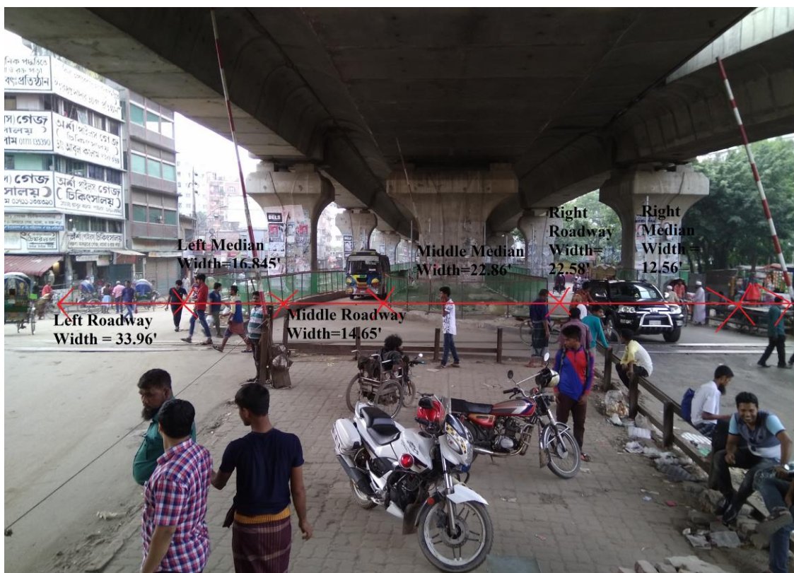
Figure 4.36: At-grade Lane width reduction at the backbone of Jatrabari-Gulistan Flyover
