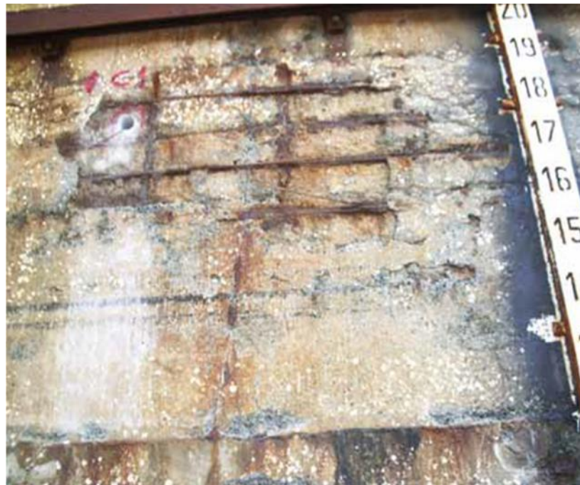
Figure 2.5: Aggression of chloride (Mapei, 2011)
