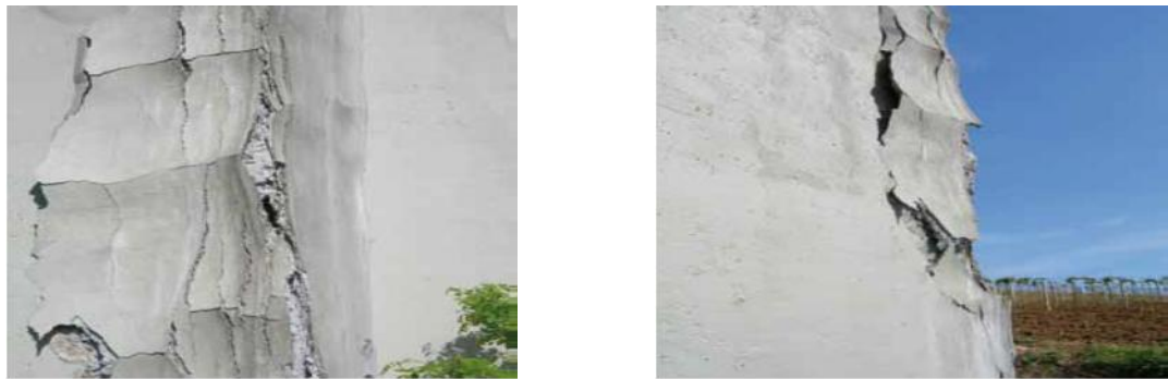
Figure 2.4: Aggression by sulfates (Mapei, 2011)
