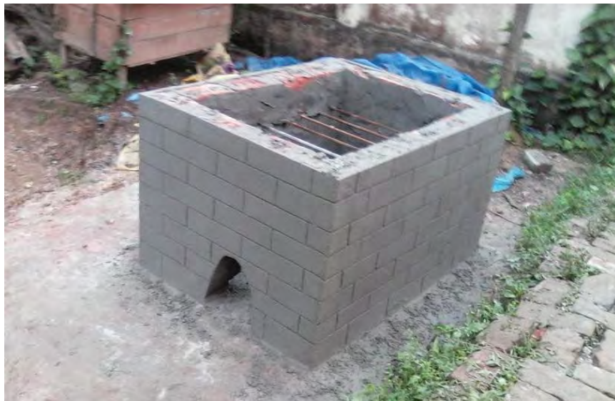
(a) Brick furnace after construction
