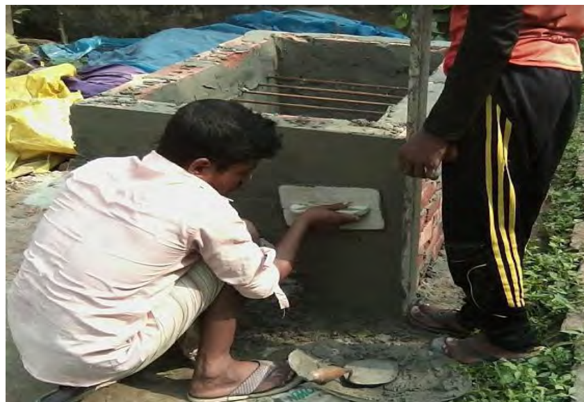
Figure A8 Making of Brick furnace
