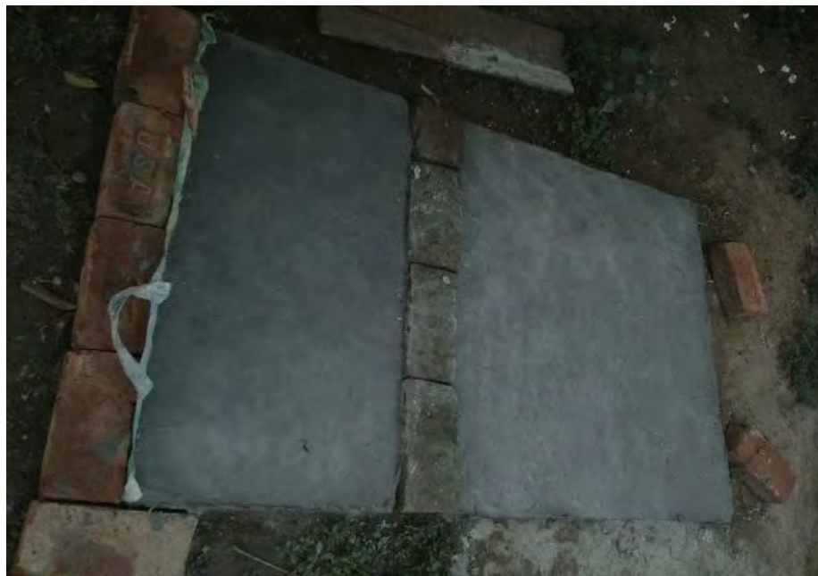
Figure A14 Collapsible slab above Brick furnace
