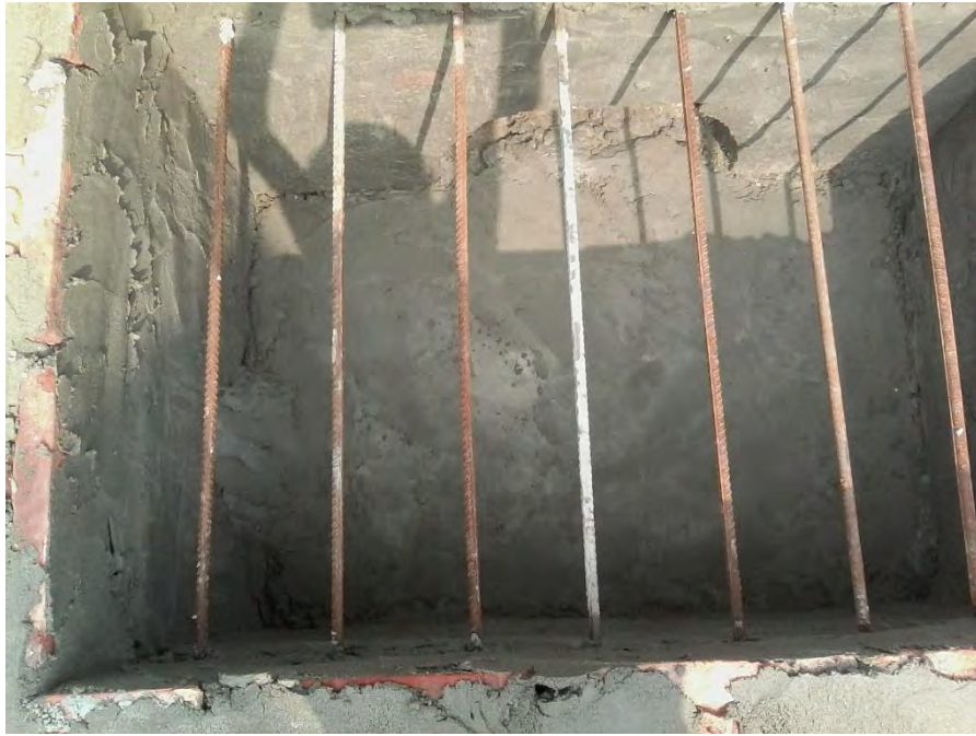
Figure A9 Top reinforcement to carry suspension bed
