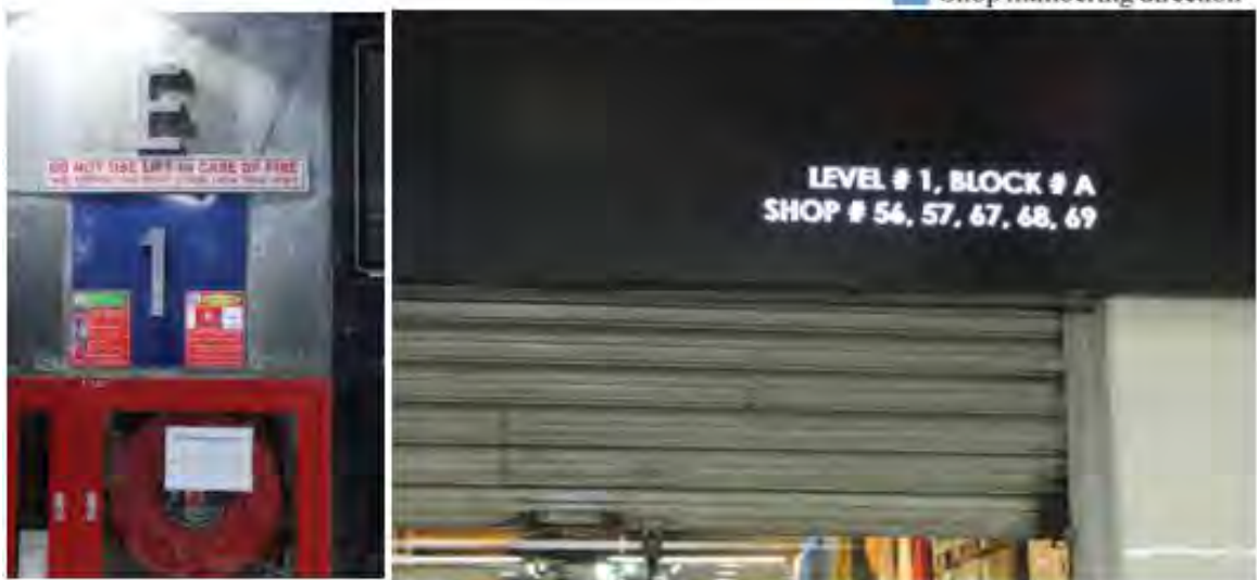
Fig 3-9: Floor identification signage (left) & shop identification signage (right)
