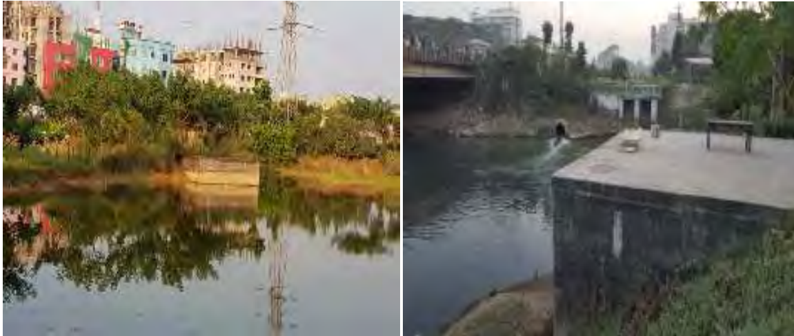
Fig 3.3: Sampling locations (pit/manhole) for collection of wastewater samples coming from the northern side (left) and Southern side (right) in Hatirjheel.
