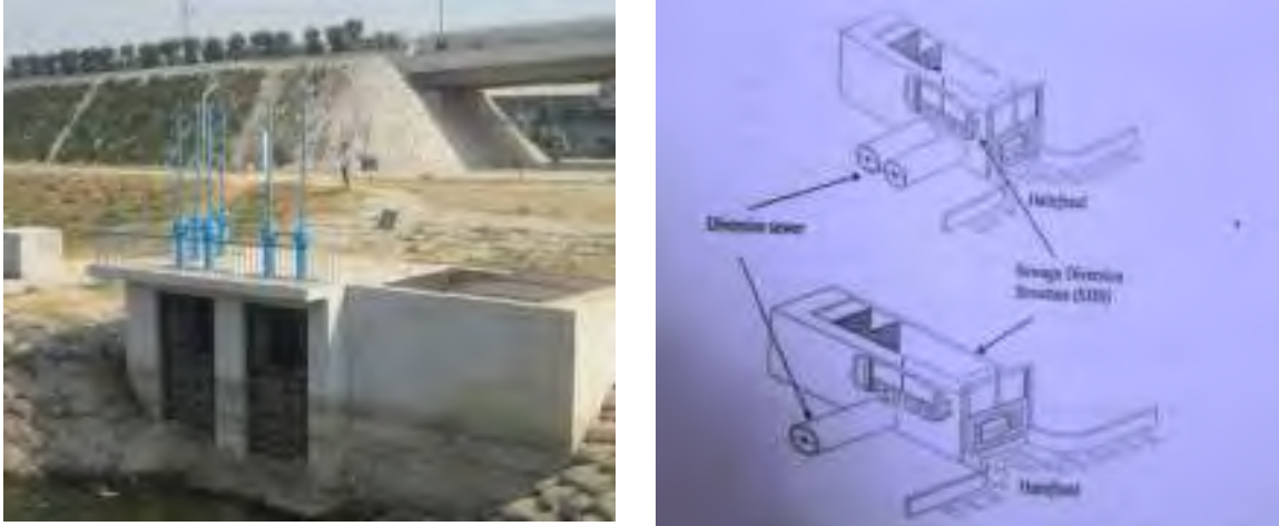
Fig 2.9: Picture of SSDS -3 in Madhubagh area in Hatirjheel (left) and typical diagram of SSDS and diversion sewers (right)
