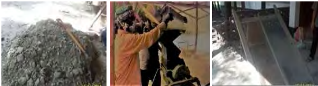
(a) Dredged soil sample (b) Soil pulverizing (c) Screened soil sample
