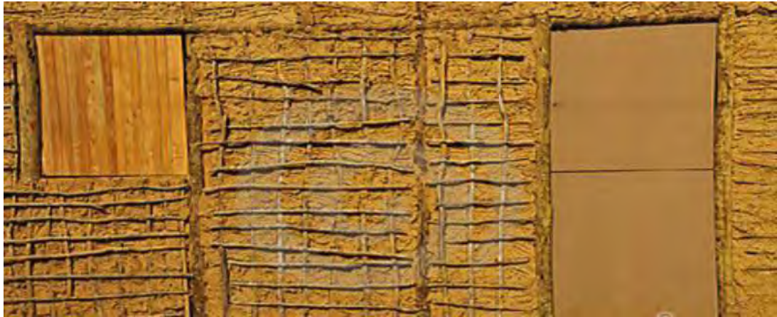
Figure 2.4: Photograph of wattle and daub (Dreamstime.com, 2010)
