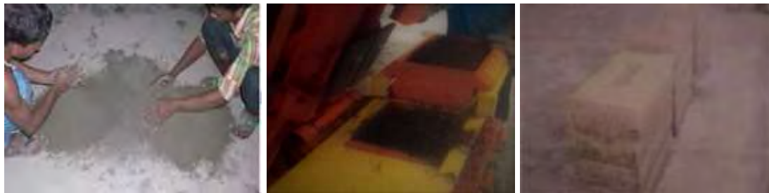
(d) Mixing cement with water (e) Filling in the mold (f) Freshly made block
