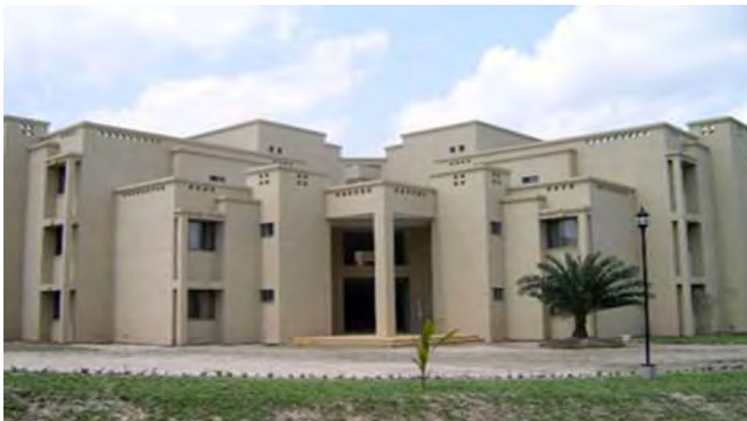
Figure 2.12: Photograph of CSEB building in CCDB HOPE CENTRE premises, Savar, Bangladesh
