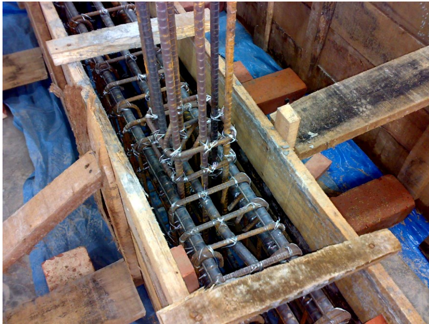
Figure 3.14 Seismic detailing of the reinforcing steel
