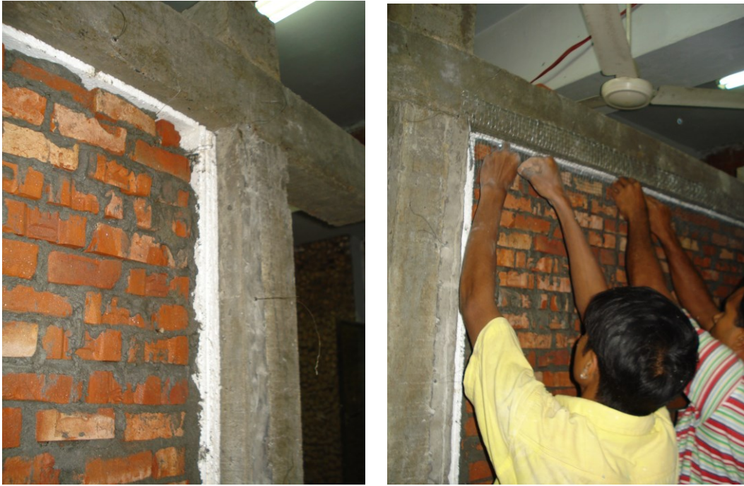
Figure 3.19 Placement of the single layer cork sheet at the infill-RC beam interface and tetra layer cork sheet at the infill-RC column interface and application of wire mesh along the interfaces
