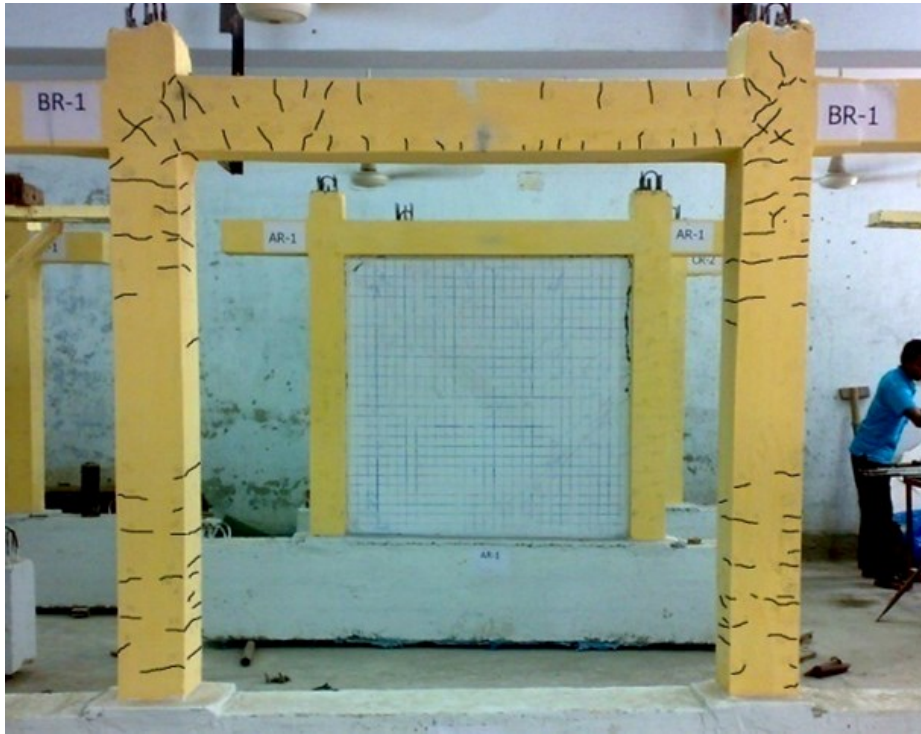
Figure 4.8(a) Crack patterns at peak load in Repaired RC Bare frame model specimen BR1
