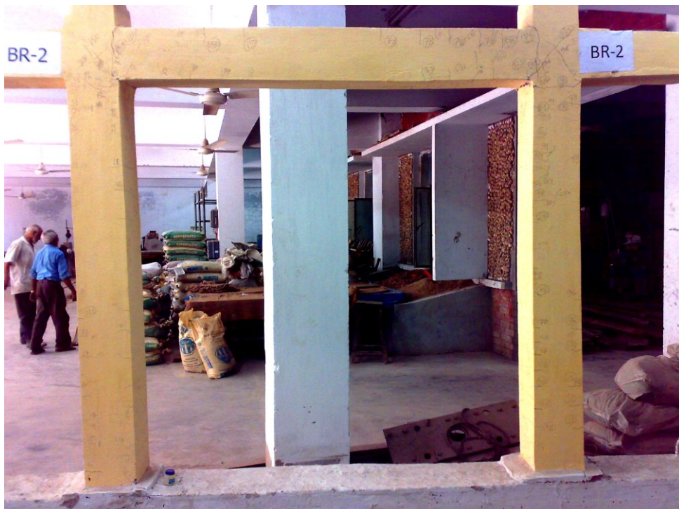
Figure 3.35 Test specimen BR2 after applying cyclic load in Test Phase-II
