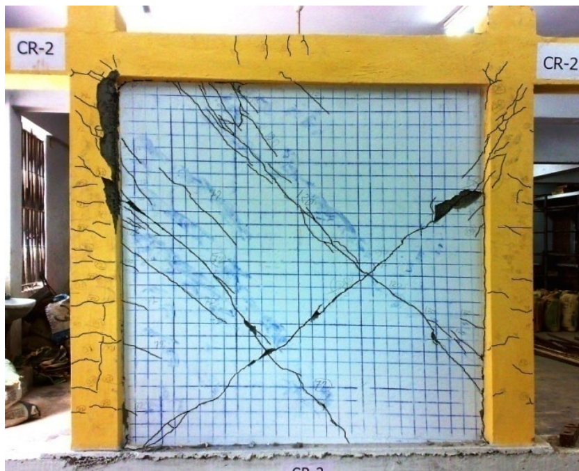
Figure 4.14(b) Crack patterns at peak load in repaired isolated infilled RC frame model specimen CR2
