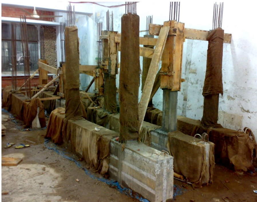
Figure 3.16 Casting of columns of the specimens
