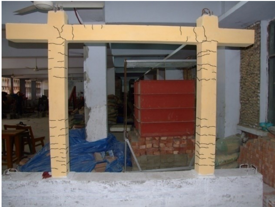
Figure 4.7(a) Crack patterns at maximum lateral load in RC Bare frame model specimen B1
