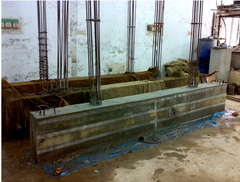
Figure 3.15 Casting of the specimens' bases in first step
