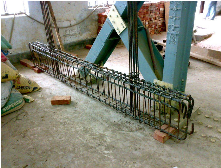
Figure 3.13 Steel casing for the specimen base
