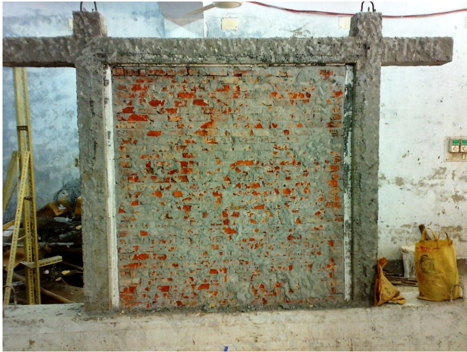
Figure 3.26 Surface cleaning of damaged specimens after chipping of plasters
