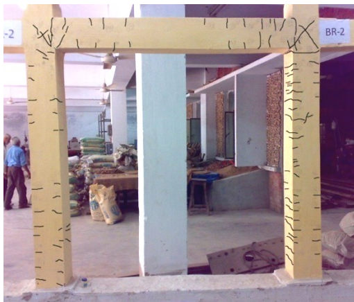
(b) Repaired bare RC frame
