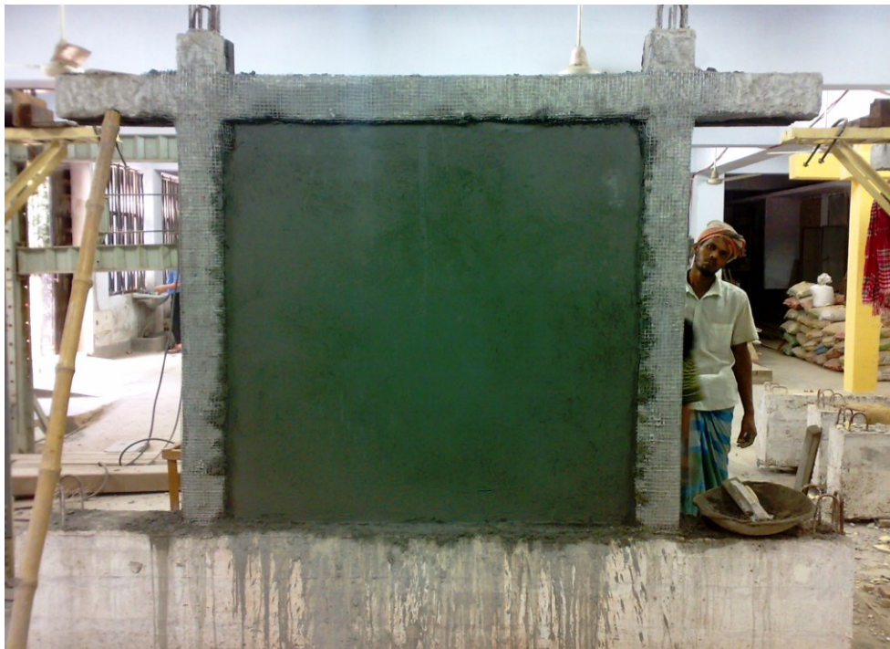
Figure 3.31 Wiremesh wrapped specimens were plastered with rich mortars
