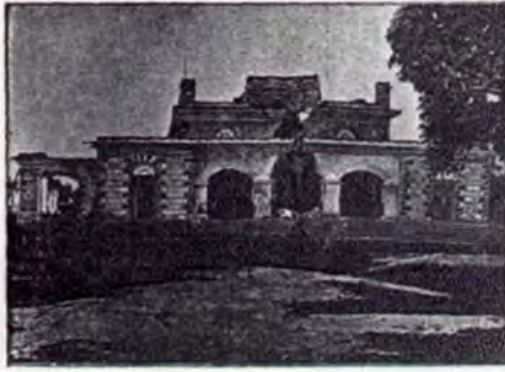
a) Damage at Rangpur, 1897 earthquake
