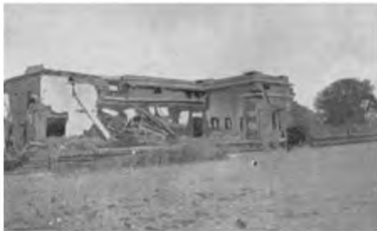
a) Sub-Divisional Officer's Bangalow, Kishorganj (Sreemangal Earthquake of July 8th, 1918)
