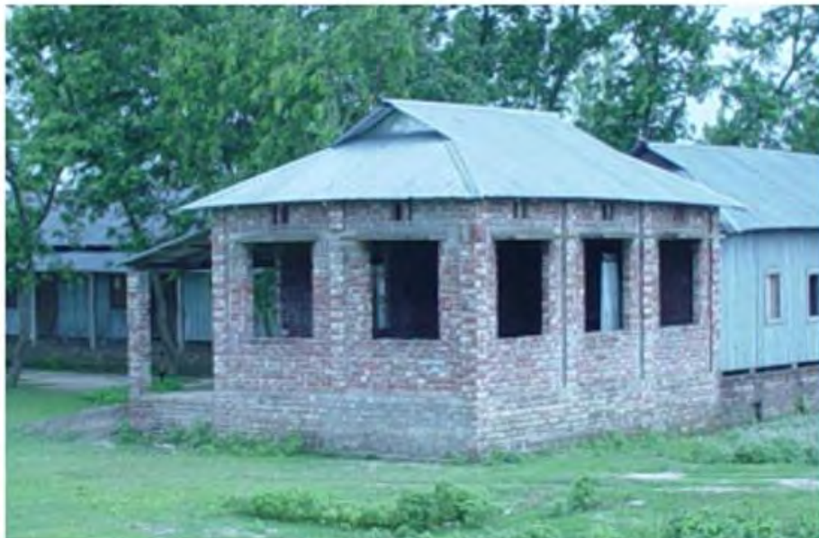
Figure 2.5 Typical Construction of Unreinforced Masonry Building (Ansary, 2003)
