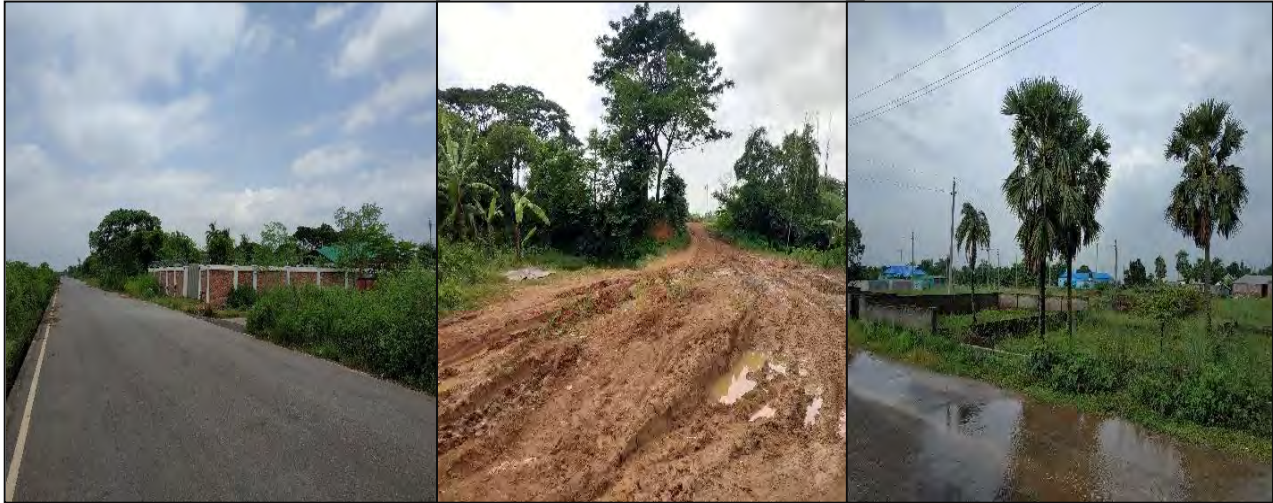
Figure 4.14: Secondary roads of PNT, Photo Taken on July 23, 2018
