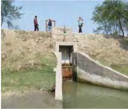
Figure A.5: Golaimari sluice
