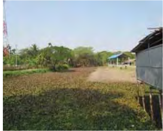
Figure A.6: Asannagar sluice covered by water hyacinths
