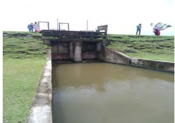
Figure A.4: Sluice gate at Telikhali New
