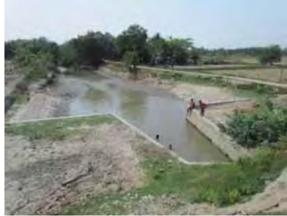
Figure A.2: Newly constructed gate inside the Bokulatola khal
