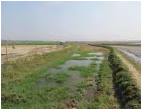
Figure A.7: Silted up course along the Aro khal
