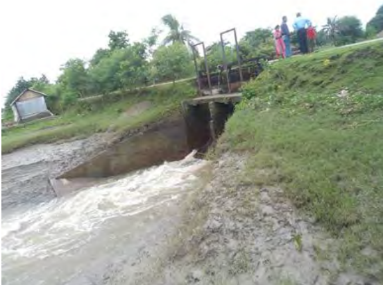
Figure A.3: Sluice gate at Telikhali Old
