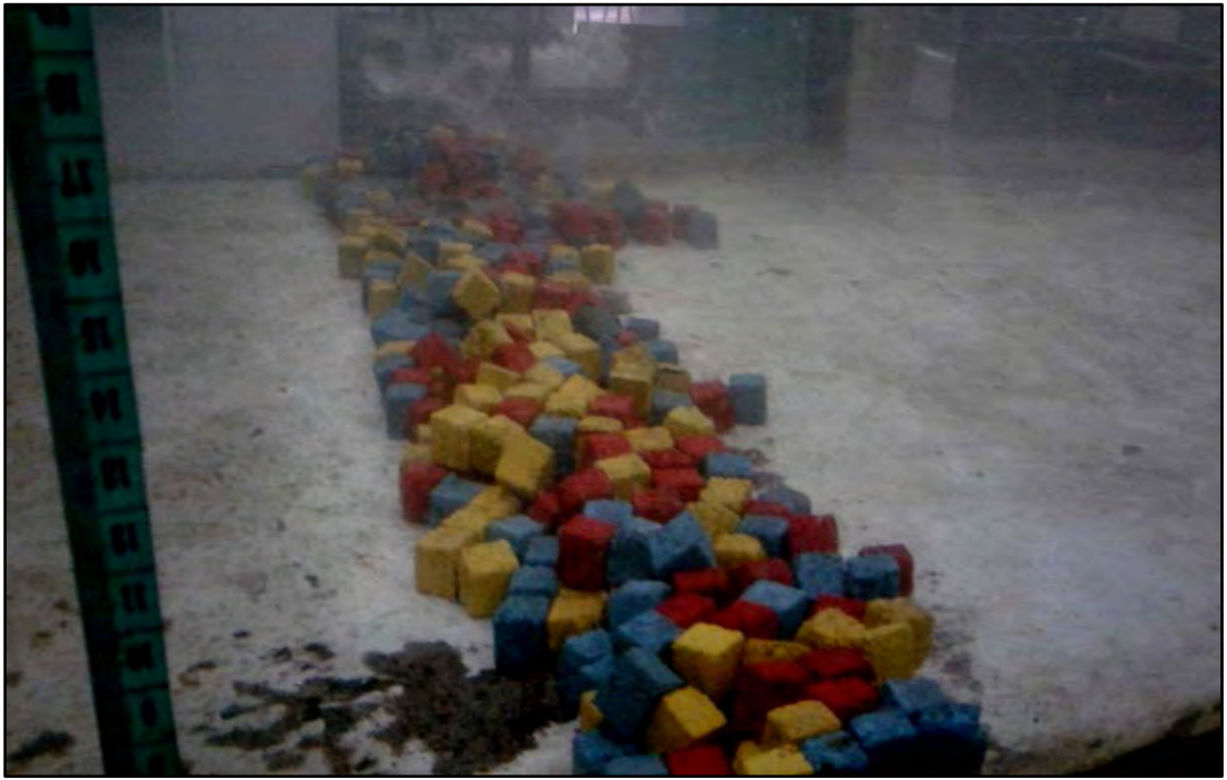
Photograph 3.7: Side view of the apron after dumping of CC blocks.
