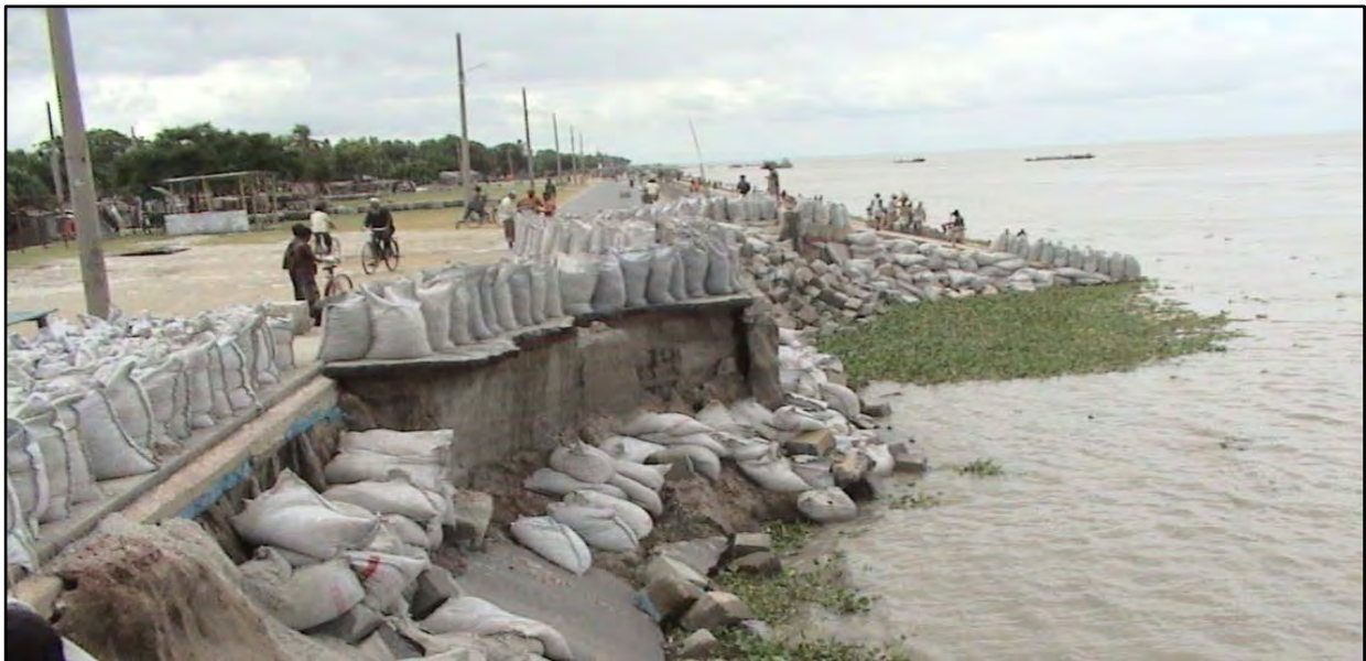
Photograph 1.1: Sand filled geobag and cc block are used to protect river bank failure.
