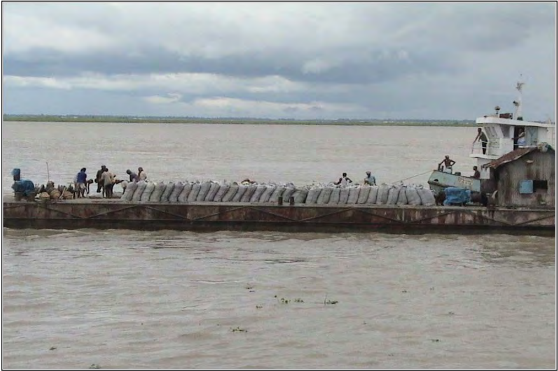
Photograph 2.1: Geobags are being dumped for toe protection.
