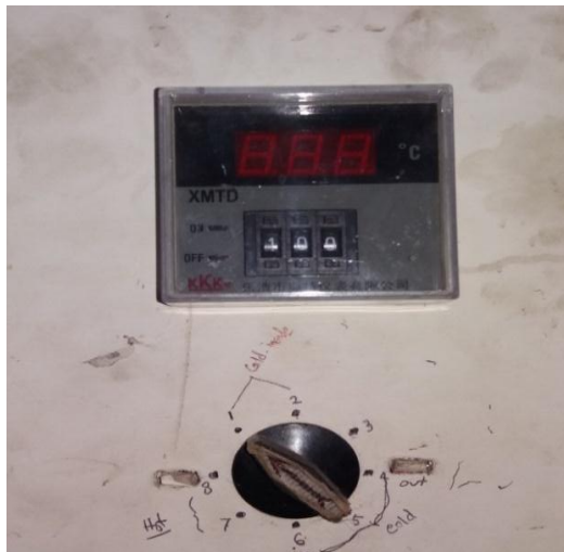
Figure 41: Measurement of temperature by thermocouple and selector switch
