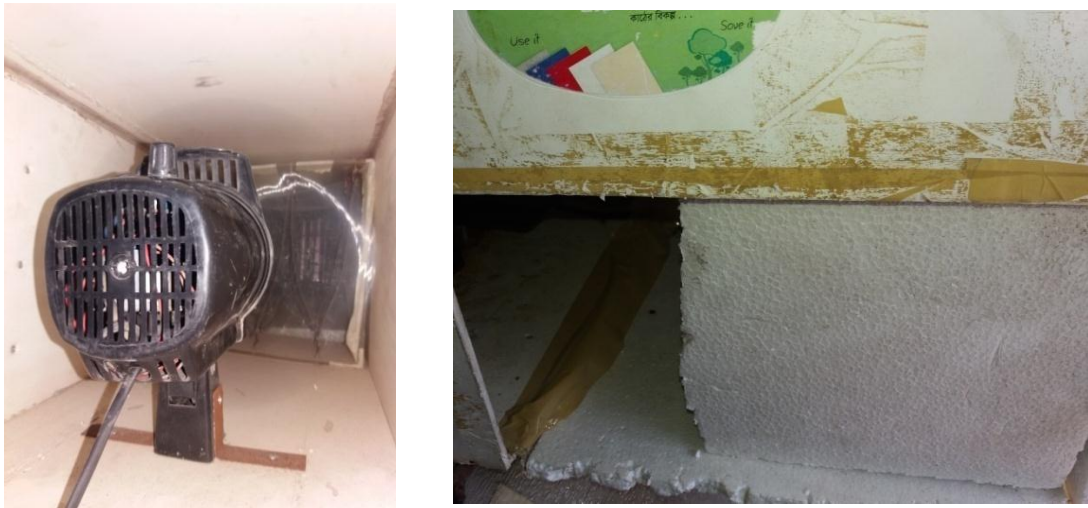
Figure 39: Regulation of hot and cold air respectively by using (a) FD fan, (b) Bypass system
