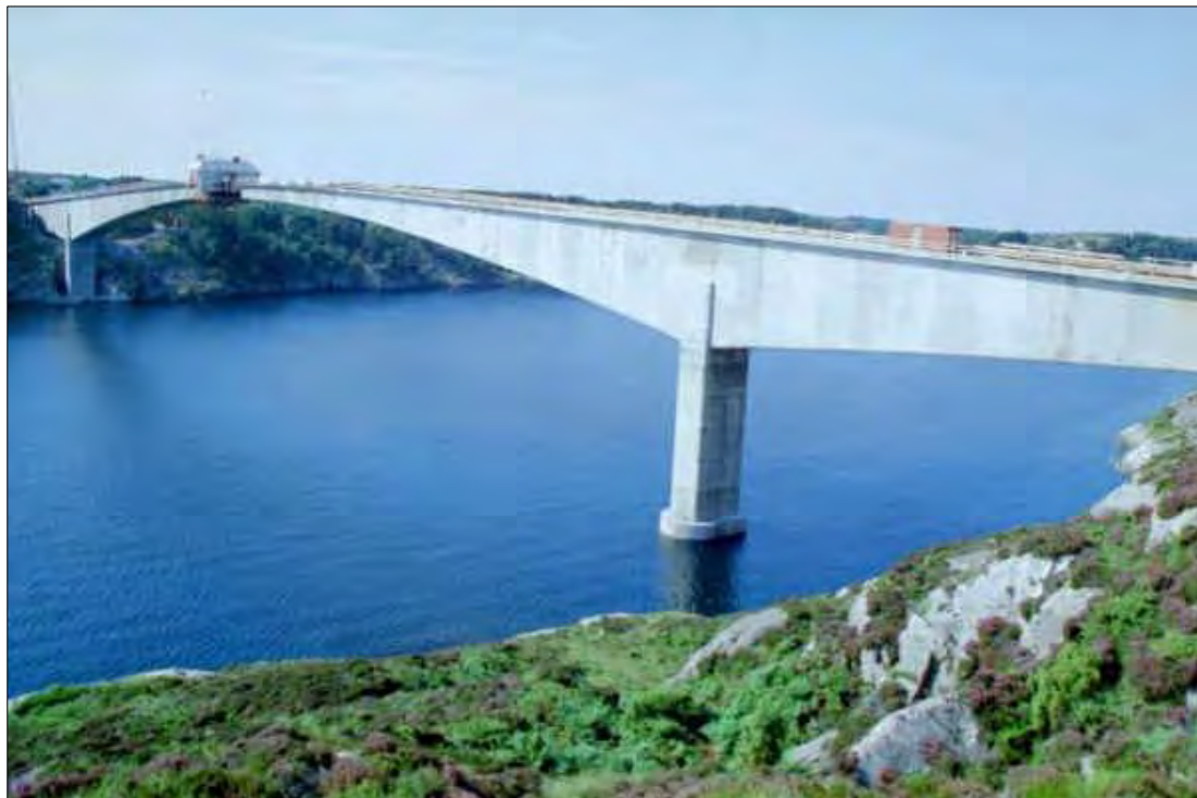
Figure 2.3: Stolmasundet bridge (Norway) (span: 301m)
