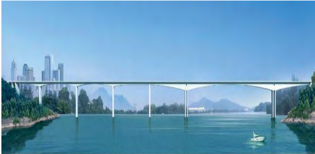
Figure 2.2: Shibanpo Yangtze bridge (China) (span: 330m) (T.Y. Lin International, 2010)
