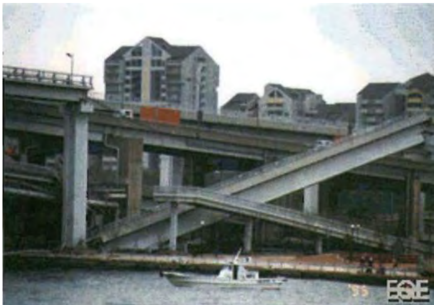
Figure 2.26: Collapsed sections of expressways in Kobe earthquake
