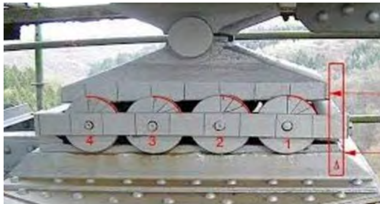
Figure 2.8: Roller bearing (Chen and Duan, 1993).
