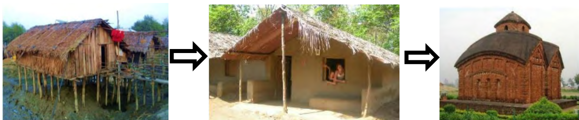
Figure 104: a. The Bamboo-woven hut on stilts. b. Thatch hut on an earth platform c. Use of Brick in Delta, “Jorbangla Mosque.”
