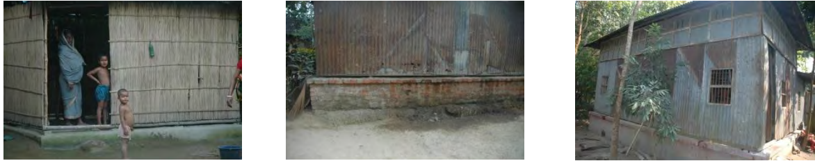
Figure 94: showing plinth from the left made of mud, semi pucca Source: (www. Google.com)
