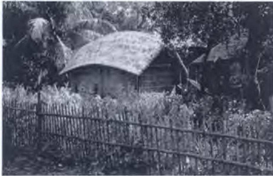
Figure 4: A traditional Bengal house form built with local material and technique Source: (Islam,2003)
