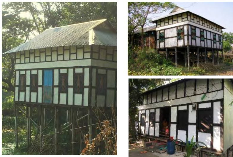
Figure 95: Transformation of traditional bamboo matting wall in the present context which is seen all over Maowa area, Dhaka
