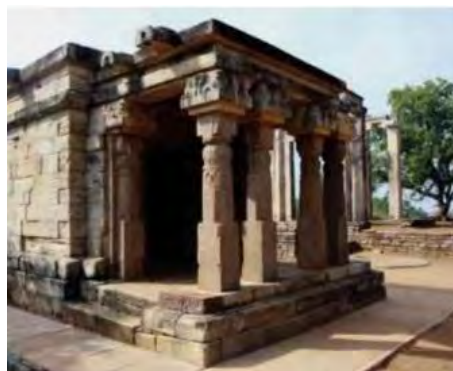
Figure 31: Temple at Sanchi showing a flat-roofed garbhagriha and mandapa, linked by a simple stepped stylobate and architrave
