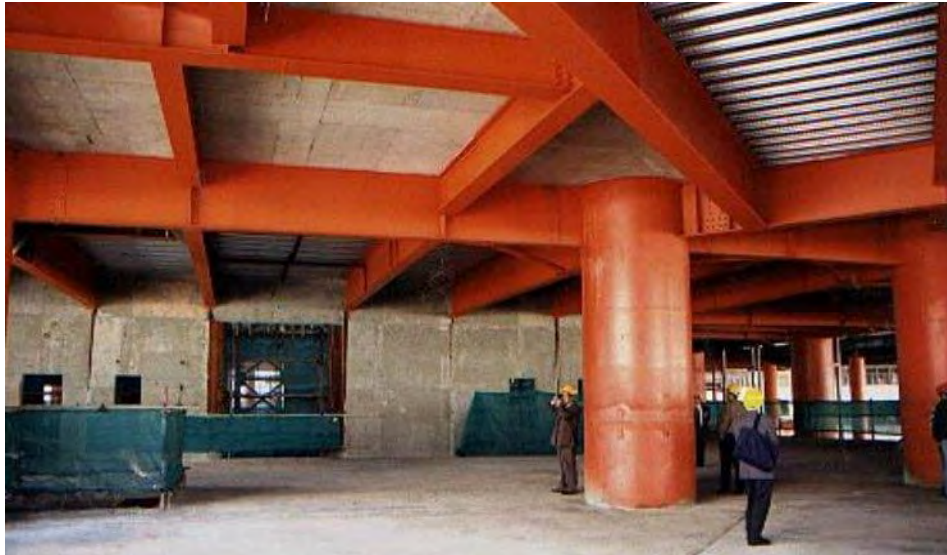
Figure 2.3 Composite steel storey system.
