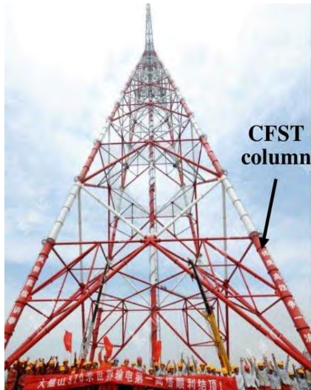
Figure 2.10 Damaoshan electricity pylon.
