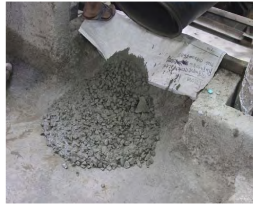
(b) Fresh Concrete
