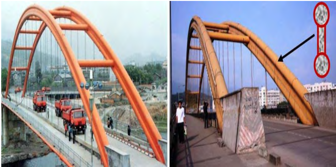
Figure 2.7 Wangcang East River Bridge.
