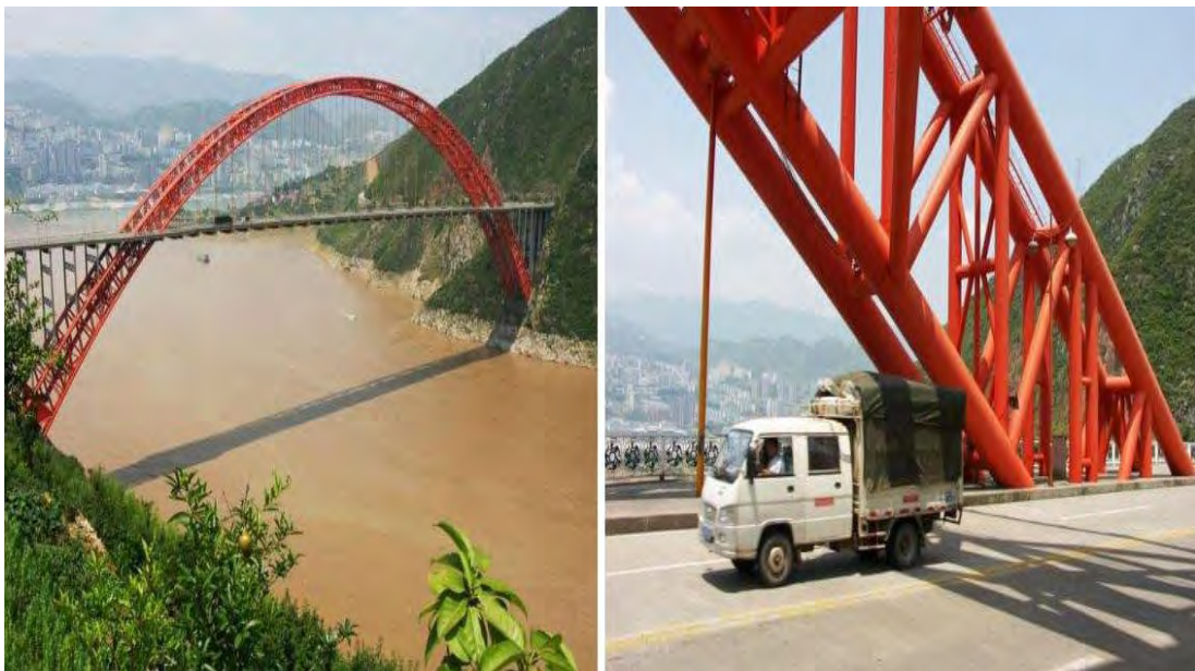
Figure 2.9 Wushan Yangtze River bridge.
