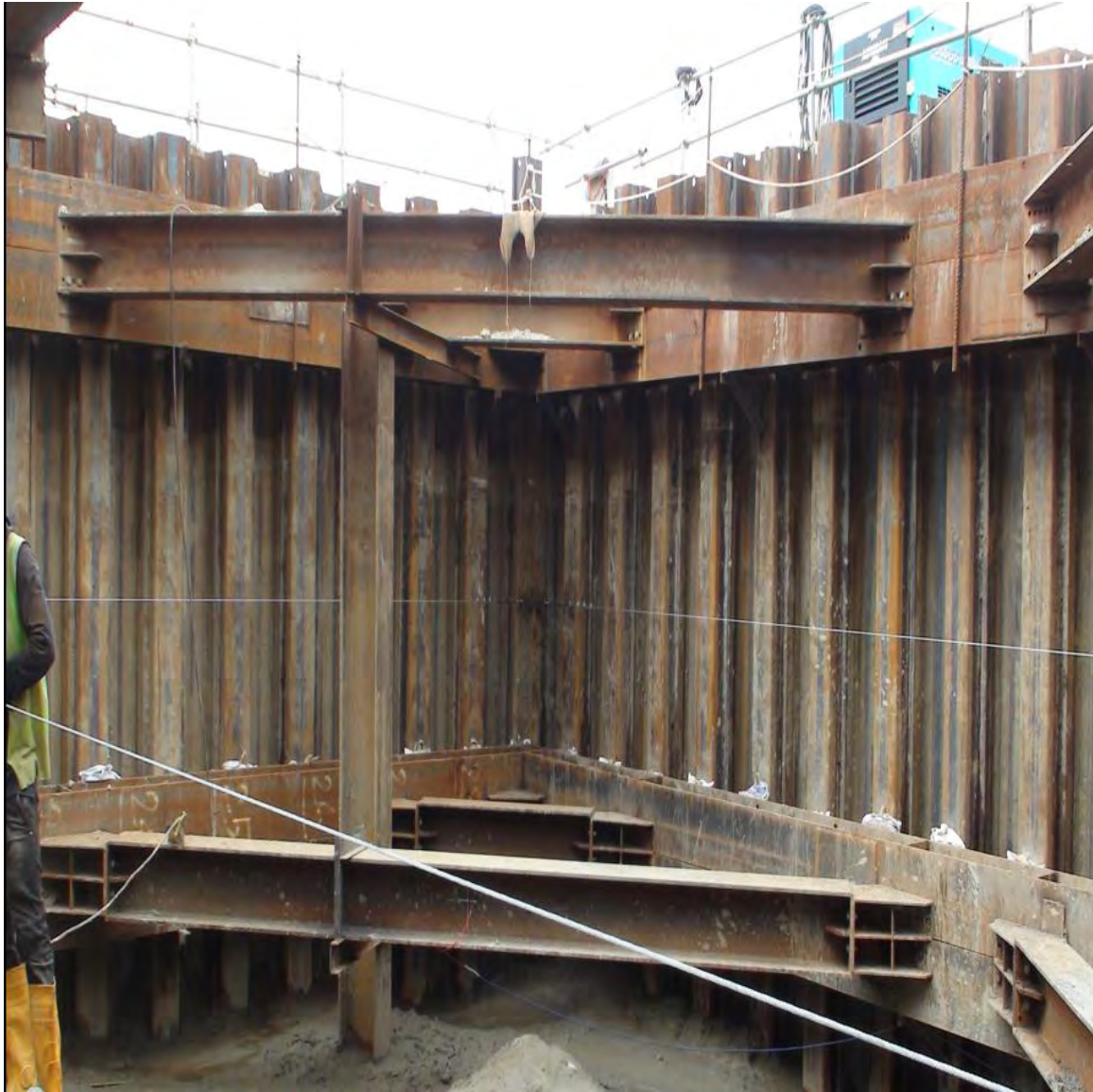
Fig. 3.12 Arrangement of struts in two levels
