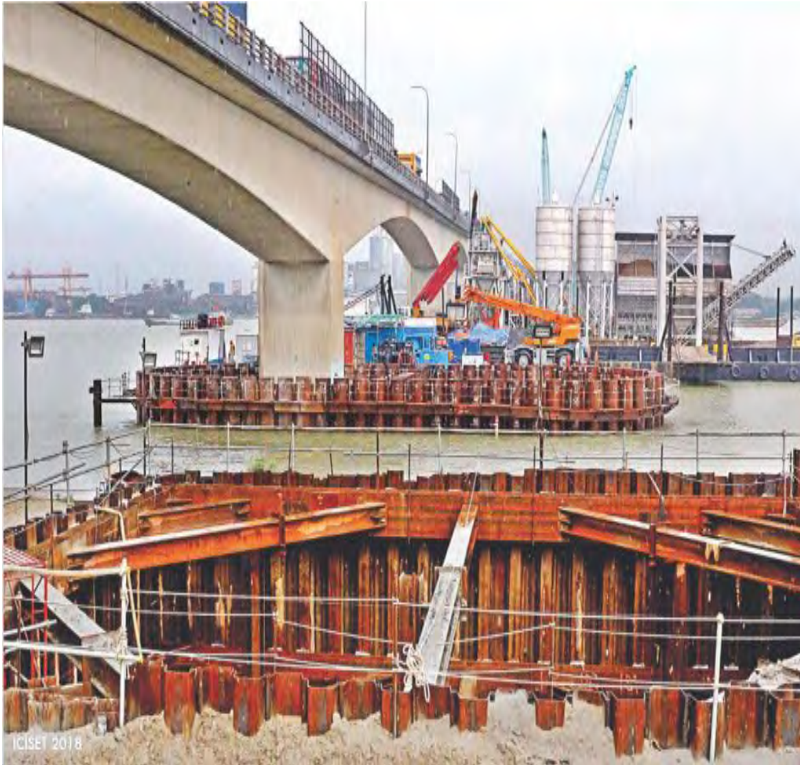
Fig. 3.11 Actual footage during construction work
