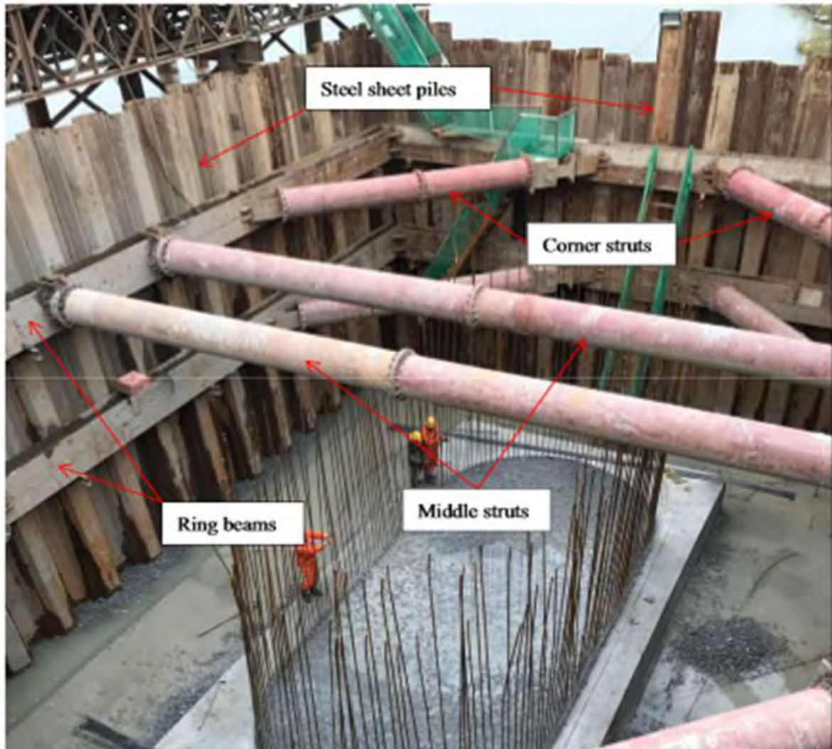
Fig. 2.21 Steel sheet piles in excavation of a bridge foundation pit.
