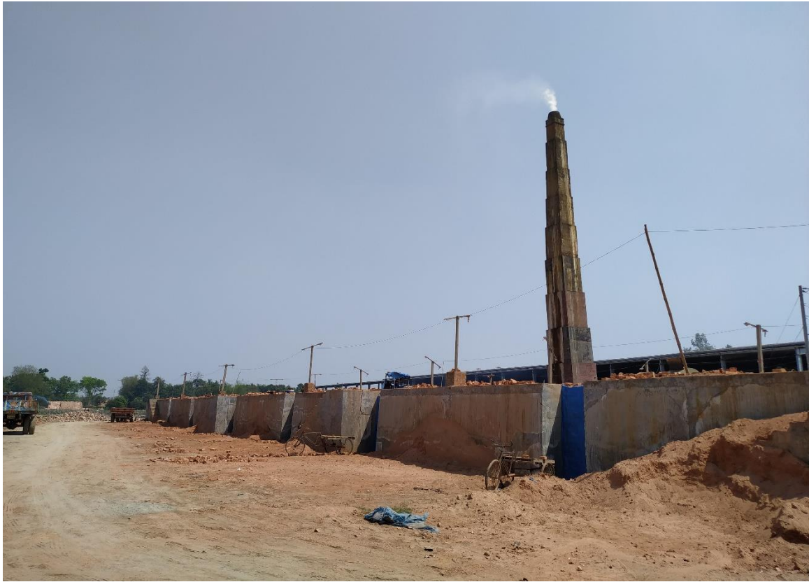
Figure 2-3: Improved Zigzag Kiln [13]
