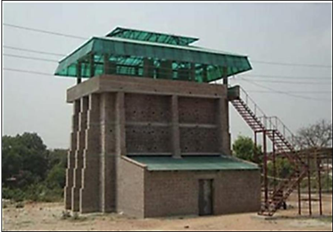
Figure 2-6: Vertical Shaft Brick Kiln (VSBK) [14]
