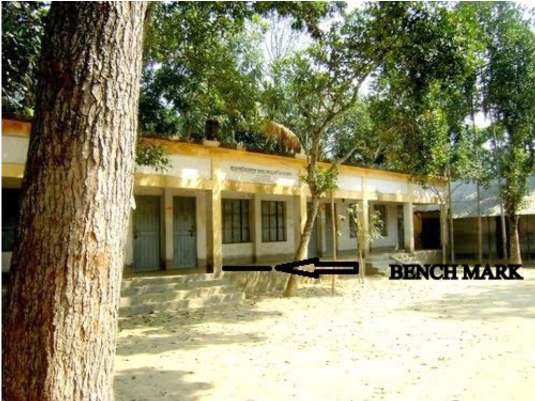
Photo 3.7: Bench Mark (BM) placed on the plinth level of the Madrasa compound by IWFM (2013).
