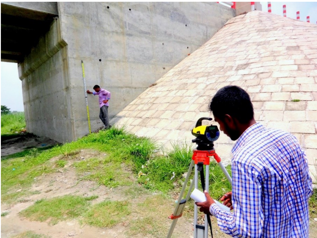
Photo 3.8: Establishment of TBM on the left abutment
