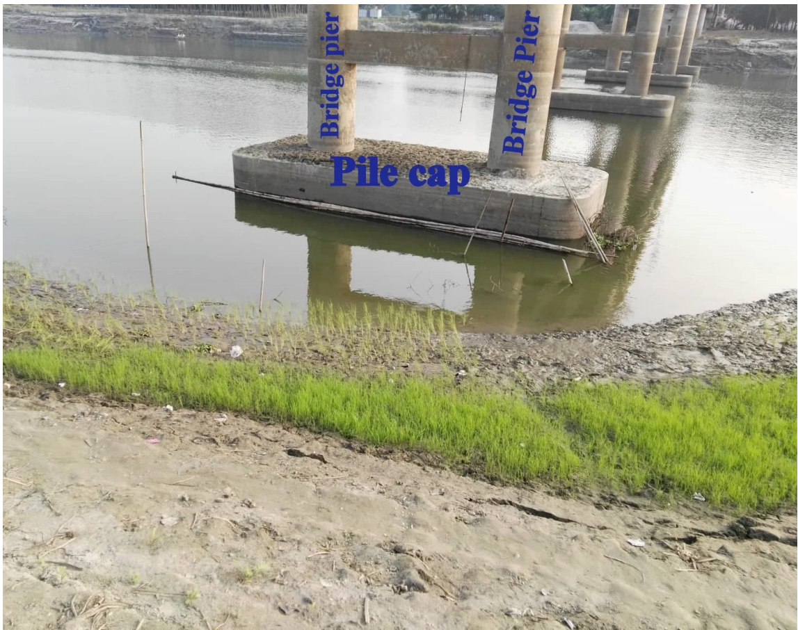
Photo 3.1: Photo showing bridge pier, pile cap, etc. (Pier no. 3).
