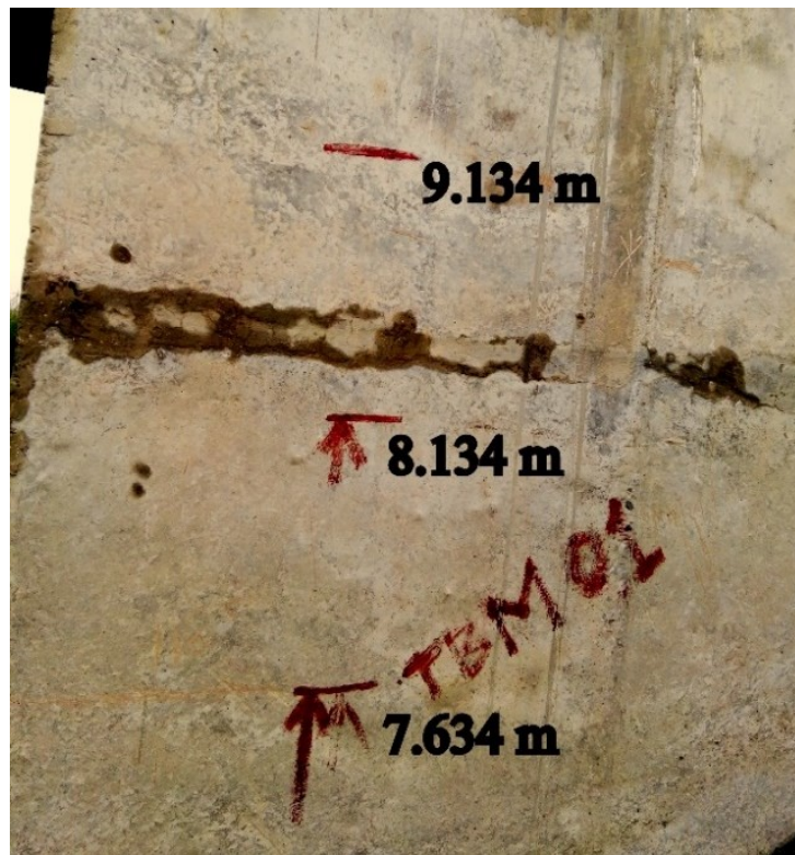
Photo 3.10: Photo showing the TBM established on the left abutment.
