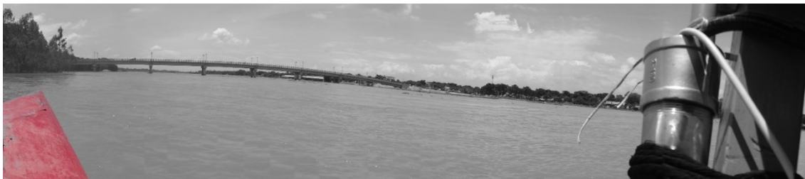
Photo 3.6: A view of the Dhaleswari Bridge taken from the boat used for bathymetric survey
