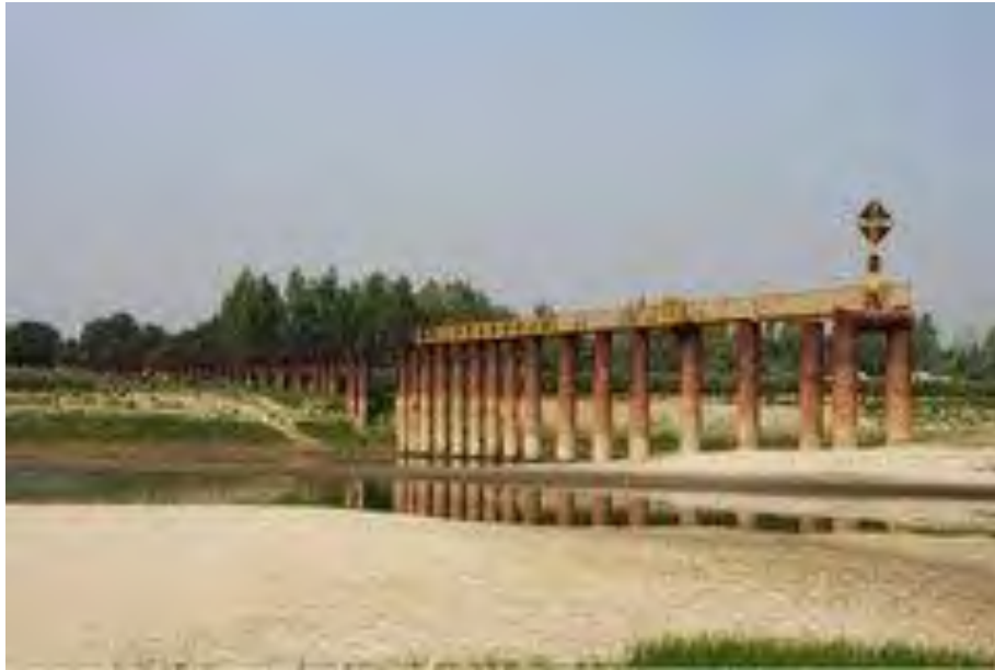
Figure 3.5: Permeable groune for Jamuna Bank protection At Kamarjani (FAP21/22)
