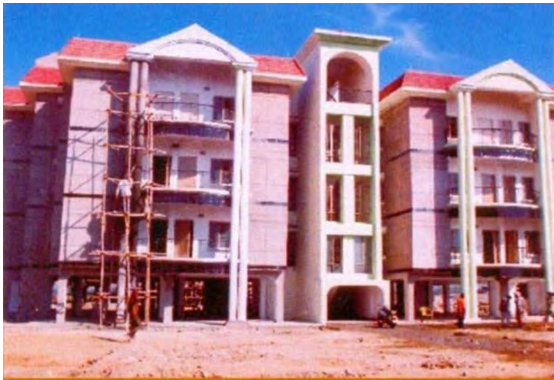
Fig. 2.13: Residential building constructed with fly-ash bricks in India
