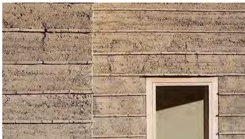
Fig. 2.5: Rammed earth (Gowda, 2016)
