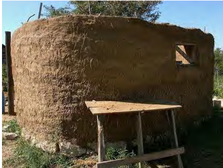
Fig. 2.2: Cob structure (Kim-Carberry, 2011)
