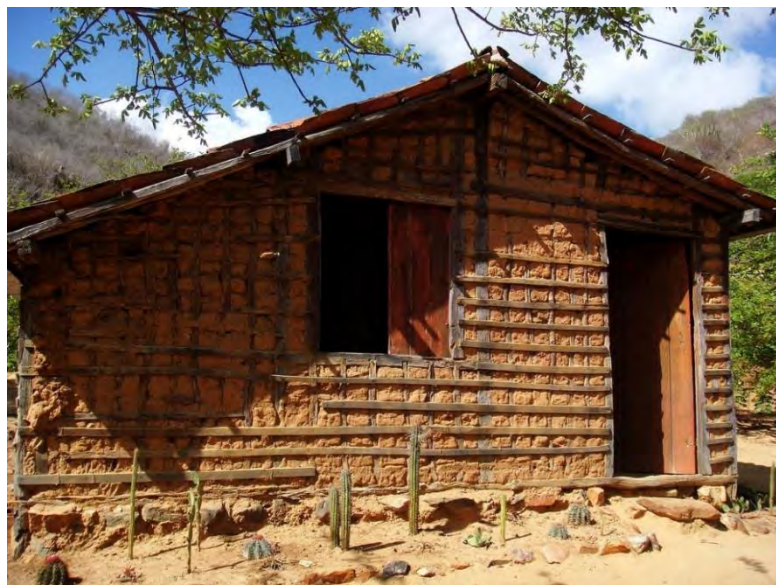
Fig. 2.3: Wattle and daub structure (Caisaem Taipa, 2018)
