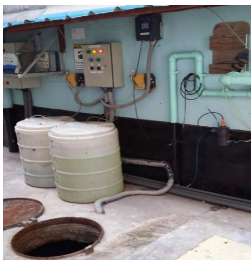
Figure 4.4: Industry's Decontamination Tank
