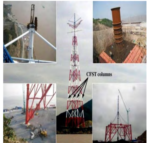
Figure 2.13 Zhoushan electricity pylon (Ren et al., 2014)
