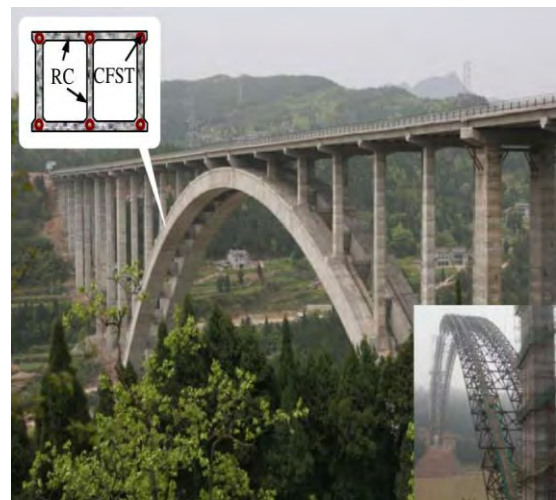
Figure 2.10 Zhaohua Jialing River Bridge (Han et al., 2014)
