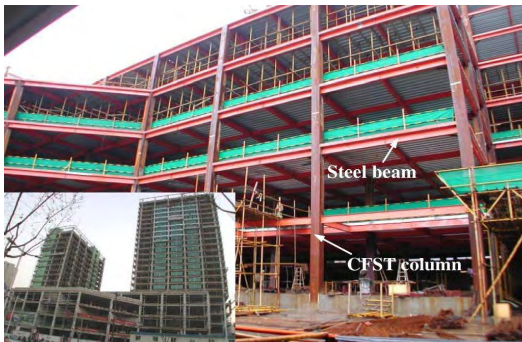
Figure 2.7 Ruifeng building in Hangzhou (Yang and Han, 2011)
