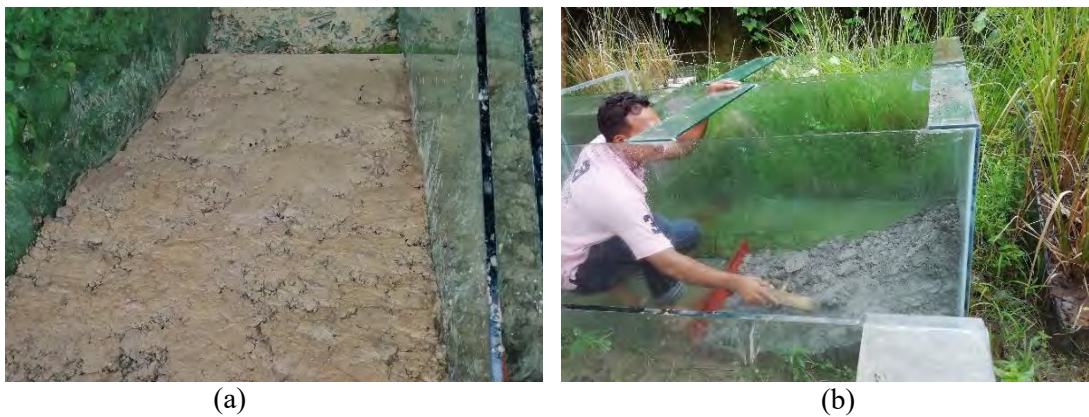
Figure 3.3: Photographs of (a) Model after Completion of Soil Filling (VM); and (b) VFM Filling by Compaction
