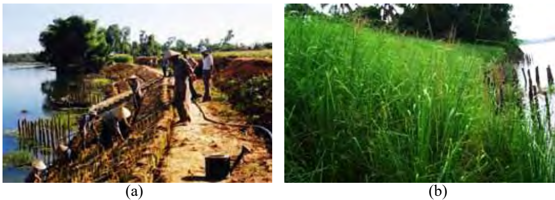
Figure 2.19: (a) Community Members Planting Vetiver; and (b) Bank Remains Intact Following the Flood Season in Quang Ngai Province, Vietnam (November 2005, funded by AusAid)
