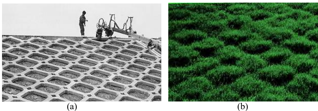
Figure 2.29: (a) Interlocking Concrete Grids Serve as Base for Plants (b) Salt Water Resistance Grass Planted on Top (USACE, 1984)
