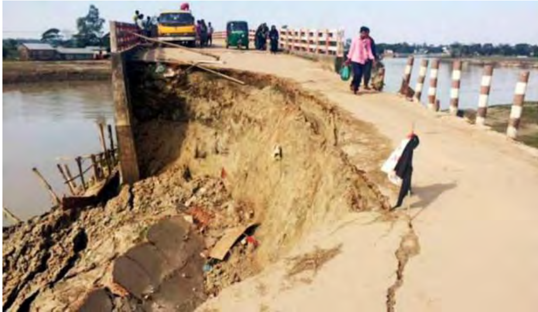
Figure 2.13: Road Slope Damage by Flood on 6 th December 2017 in Jagannathpur Upazila, Sunamganj (The Daily Star, 2018)
