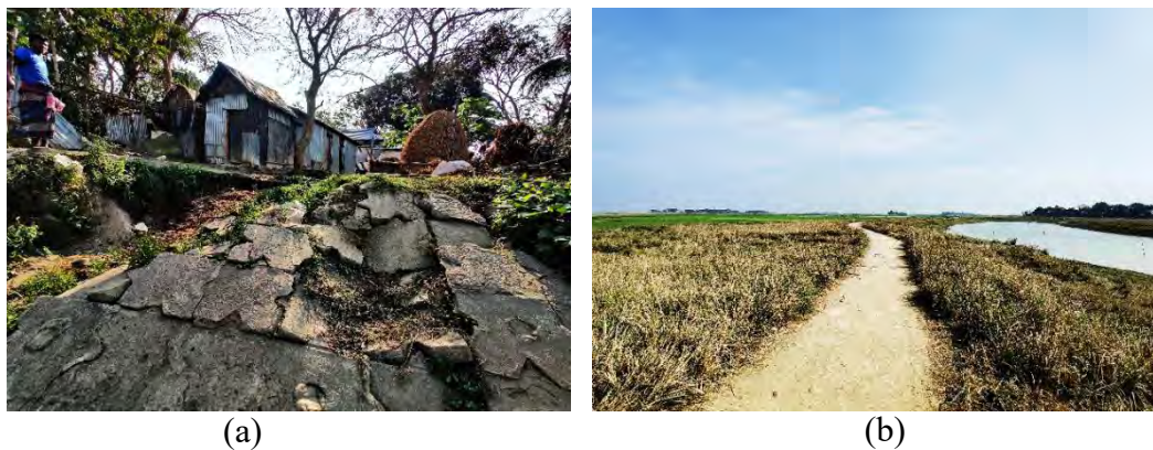
Figure 4.28: Site Condition of Hayatpur, Khaliajuri, Netrokona; (a) Slope Condition of the Village Island; (b) Well Condition of the Vetiver Source
