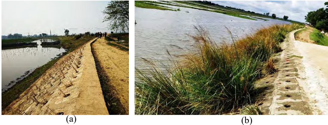
Figure 4.25: Photographs of Protection Type III at Vatipara, Baniachong, Habiganj; (a) 20 Days after Plantation (26 th January 2019); and (b) After Facing One Flood (11 th November 2019)
