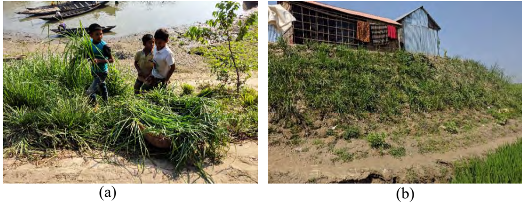
Figure 4.27: (a) Trimmed Vetiver Selling for Fuel and Fodder; (b) Slope Protection with Vetiver by Villagers in Kamalpur, Nikli, Kishoreganj
