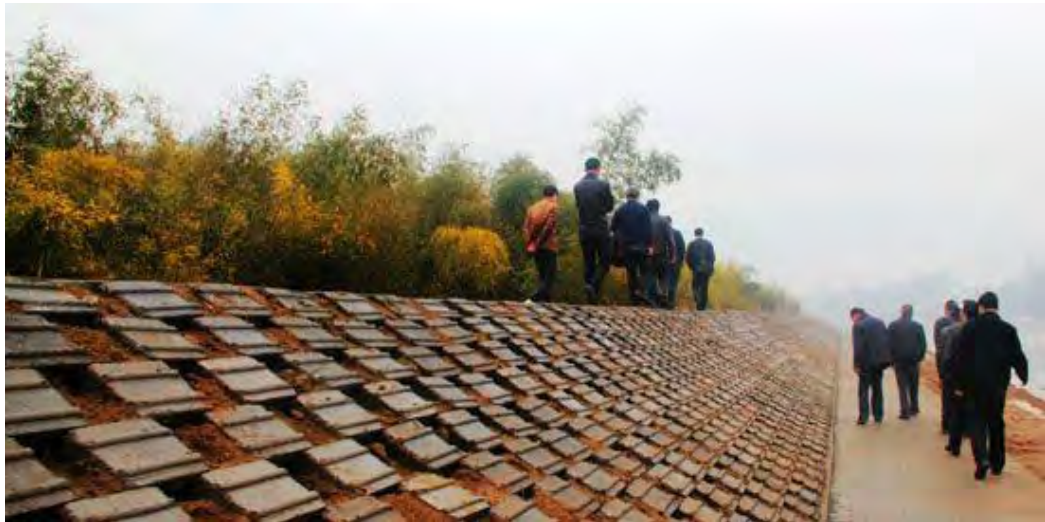
Figure 2.30: Ecological Revetment Built in Qiyun Mountain, China (2013)
