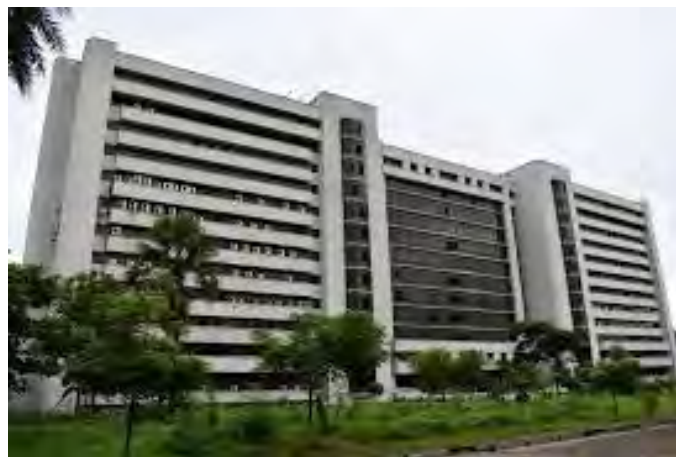
Figure 4.9 BUET ECE building
