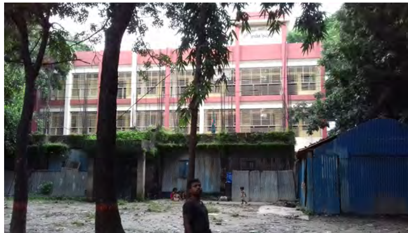
Figure 3.10 Case school building Paikpara Government Staff Quarter Primary School
