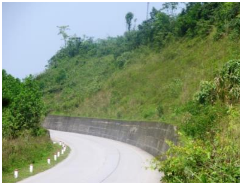
Figure 2.14: Vetiver system along Ho Chi Minh Highway, Vietnam (Source: Xuan, 2014)
