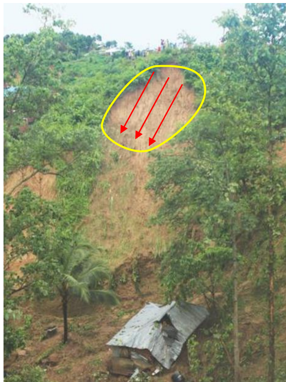
Figure 2.12: Probable slide location and damaged house in Rangamati (Source: The Daily Star, June 19, 2017)
