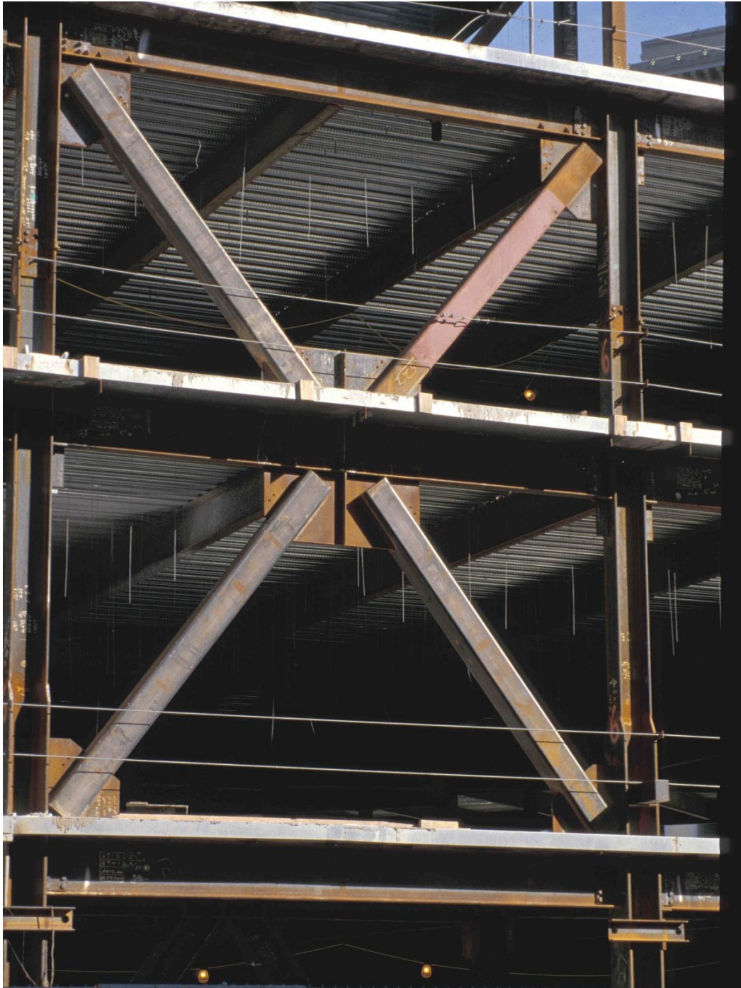
Fig. 2.2: Concentrically Braced Frame (CBF) (Engelhardt 2007)
