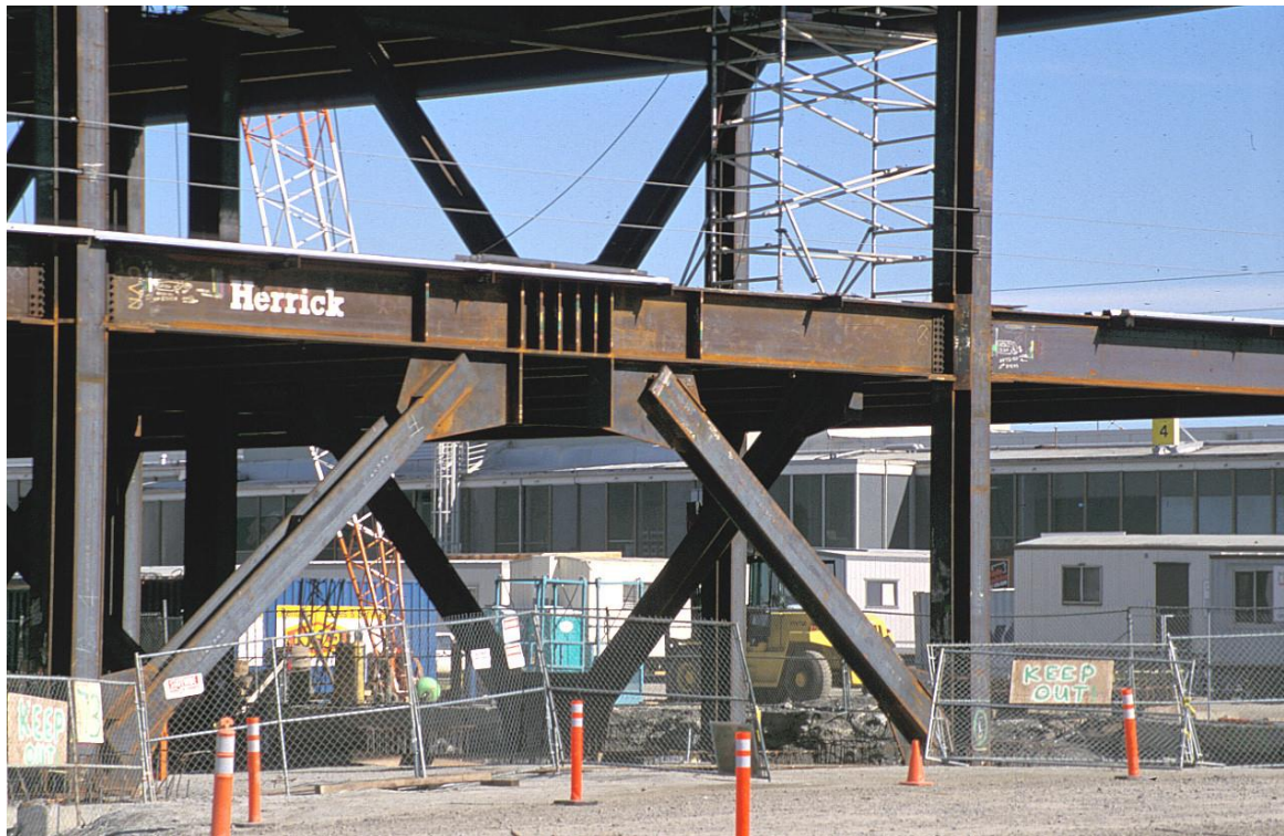
Fig. 2.3: Eccentrically Braced Frame (EBF) (Engelhardt 2007)
