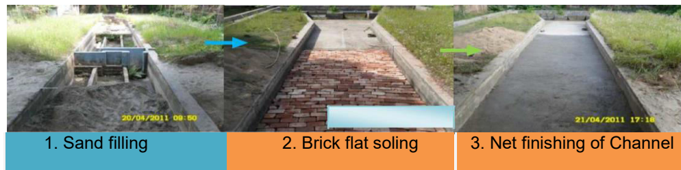
Figure 3.9: Construction Stage of Meandering Channel
