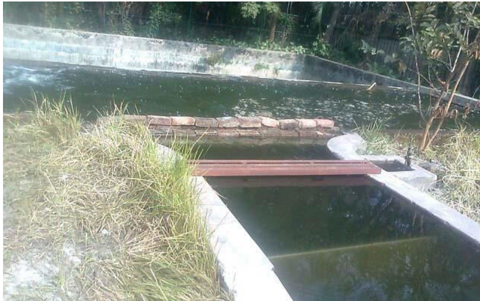
Figure 3.2: Upstream reservoirs, the approach channel including the sharp crested weir
