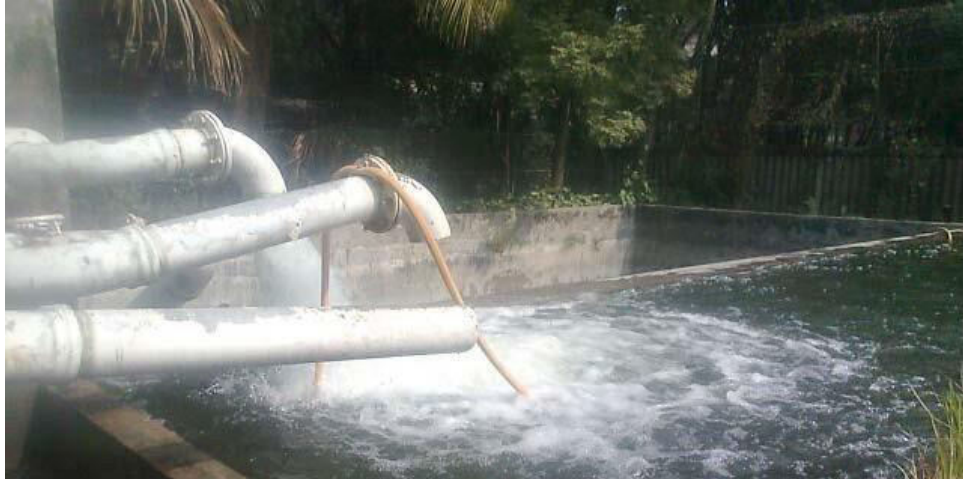
Figure 3.5: Water supply system from the centrifugal pump
