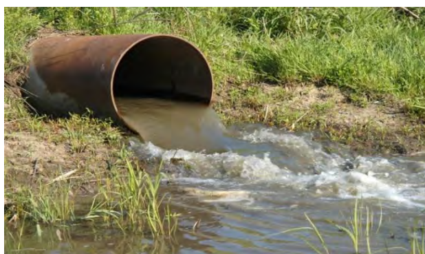
Waste disposal through drainage systems
