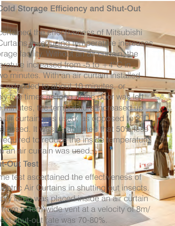
Fig. 1.14 (a) Air curtain installed in shop front, photo from Thermoscreens air curtains, (b) Air curtain's Shut-out Functions, photo from Mitsubishi Electric air curtains.
