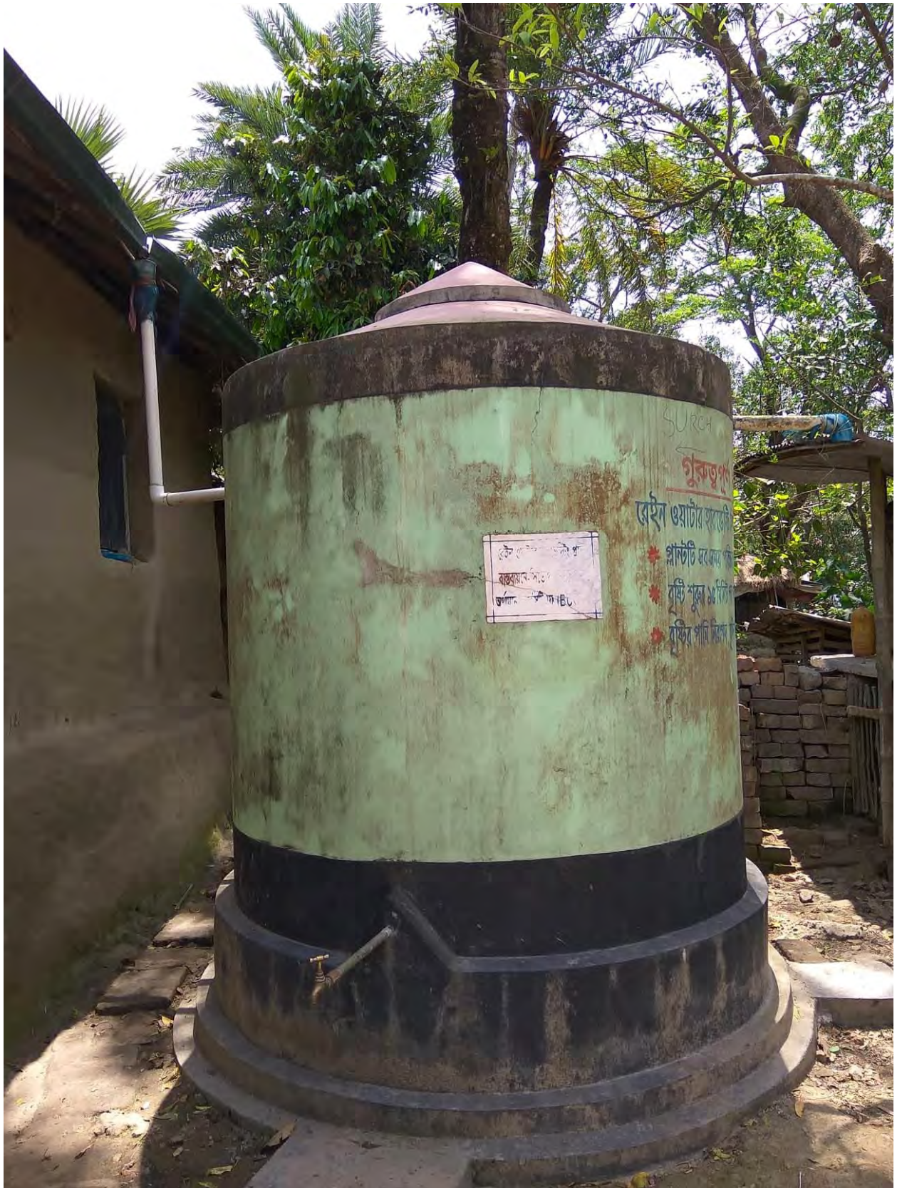
Photo 7.5: A typical setup for rainwater harvesting in a household in Pankhali
