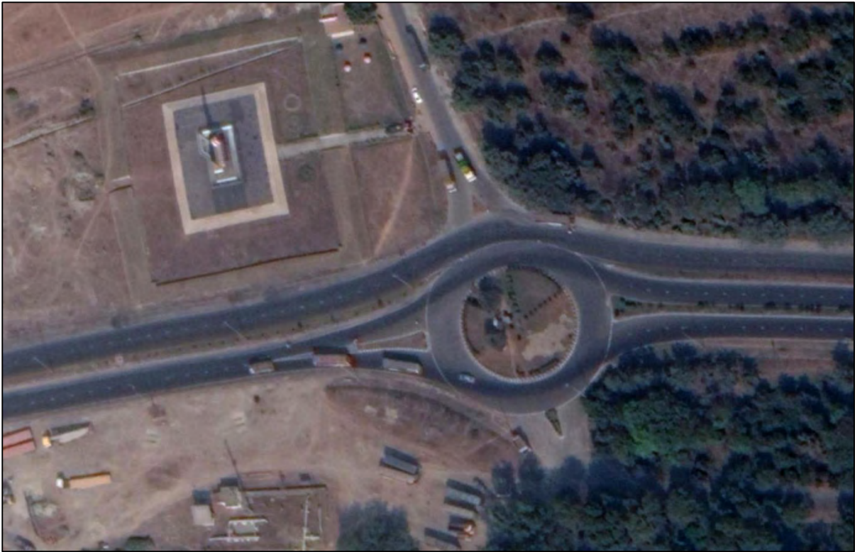
Figure 3.3 Google Earth location image of Bangabandhu bridge west roundabout
