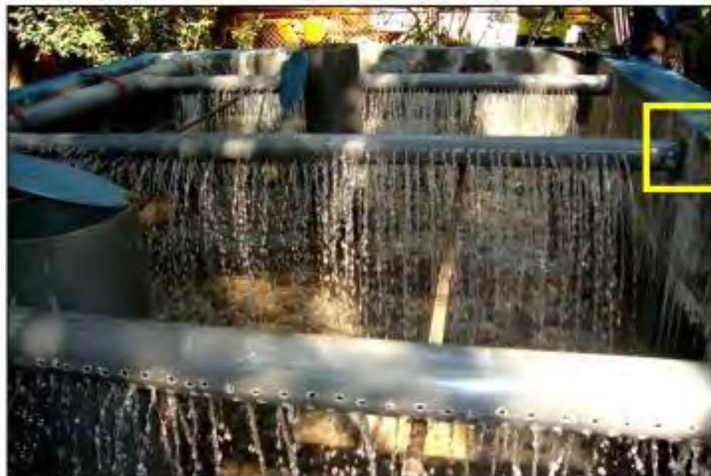
Figure 6.4: Release of Rainwater through Shower Pipe (Source: DWASA, 2018)
