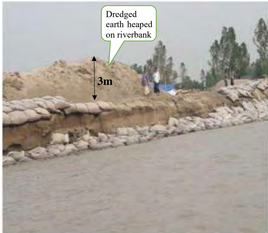
Figure 5.62: Surcharge load kept over riverbank after dredging
