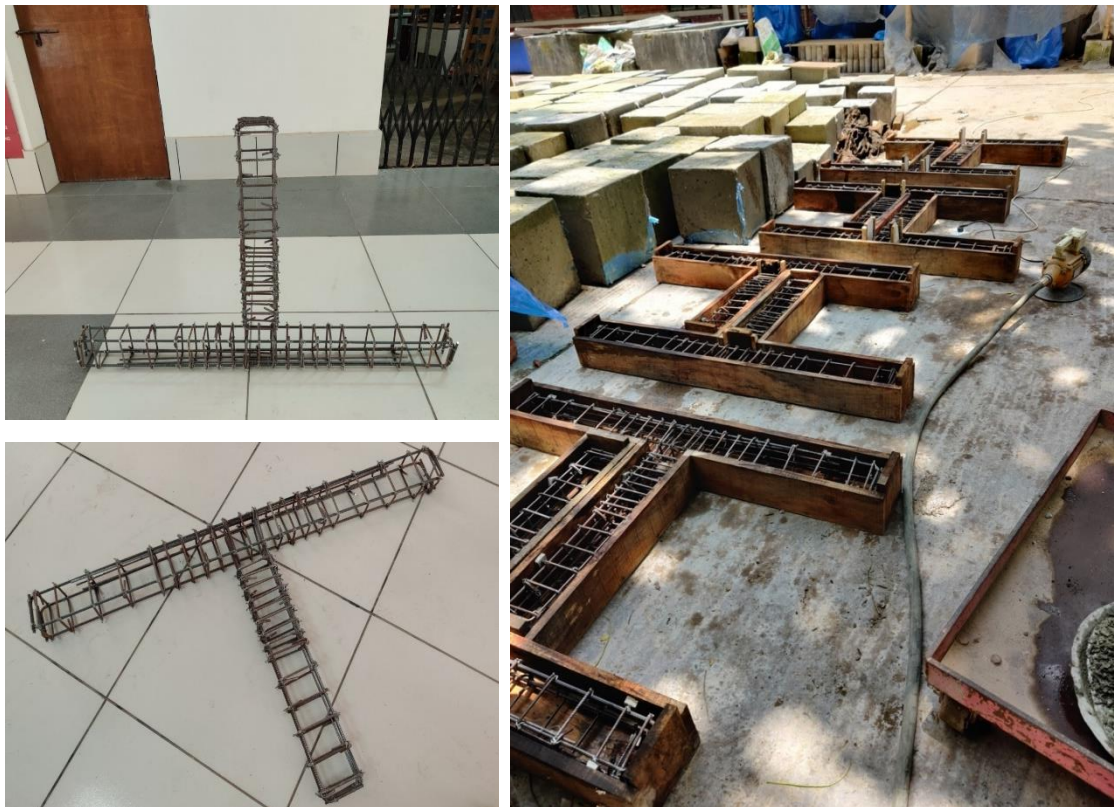
Figure 3.20: Preparation of reinforcements
