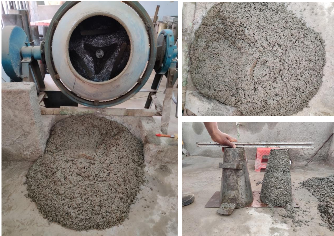
Figure 3.21: Preparation of concrete mix
