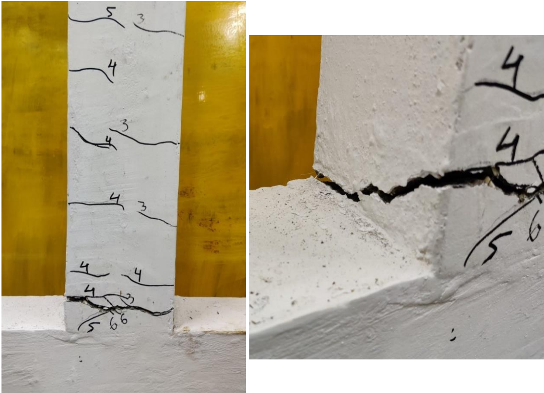
Figure 4.1: (a) Cracks in specimen 1-SS-C1 (b) Failure zone of specimen 1-SS-C1
