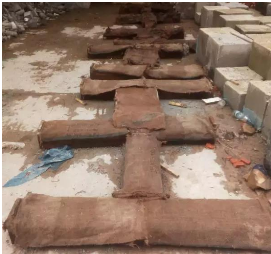
Figure 3.24: Curing of concrete
