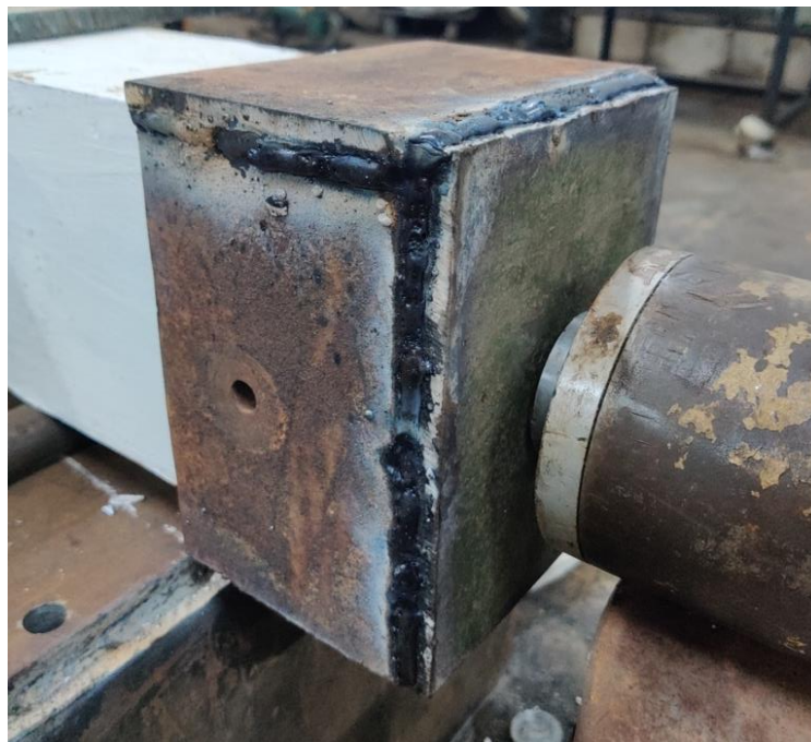
Figure 3.27: Customized steel capping at column ends
