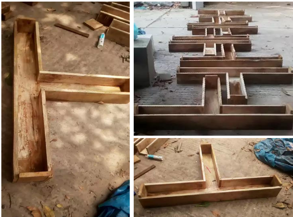
Figure 3.19: Preparation of formworks
