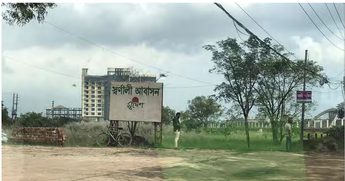
Photo: Project View of Shornali Abashon, Swadesh Properties Ltd. Source: Survey of the Shornali Abashon
