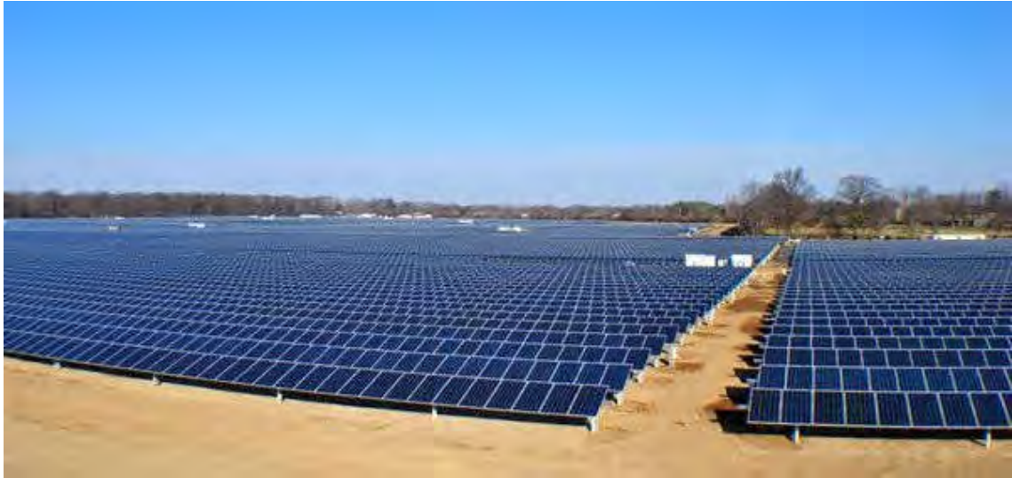
Figure 2.2 Fixed tilt mounting system
