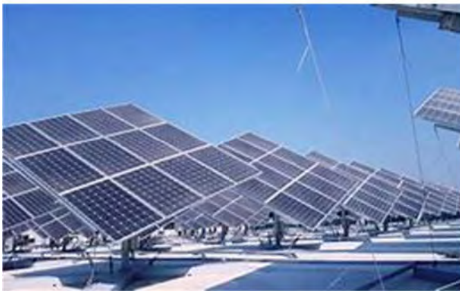
Figure 2.5 Dual axis tracker
