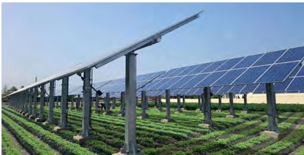
Figure 2.3 Horizontal single axis tracker
