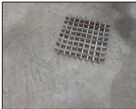
(i) Formwork of C.C. block
