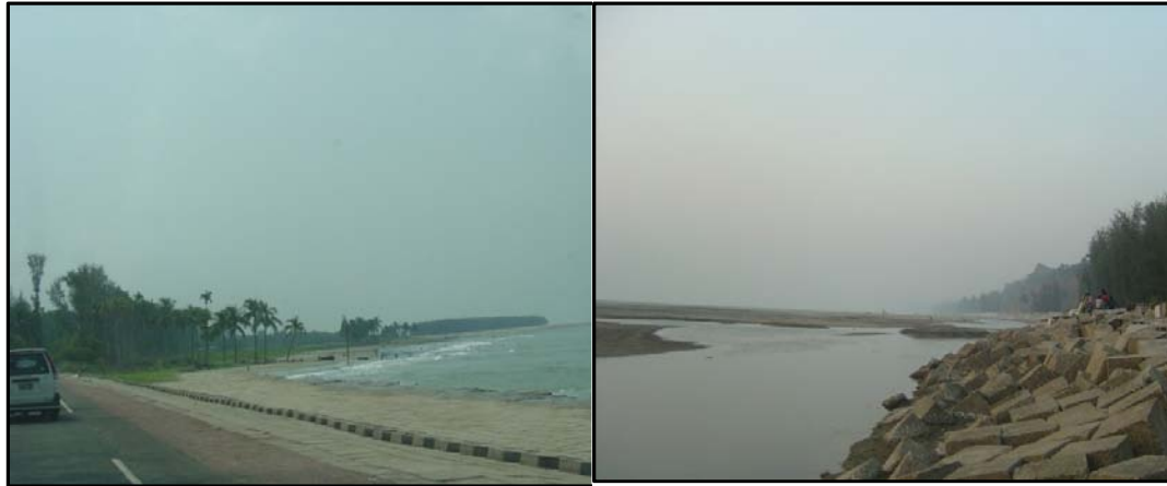
Figure 1.3: C.C. block revetment on Marine drive (2008) (© M. A. Rahman)
