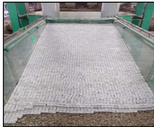
(viii) Constructed Revetment (top view)
