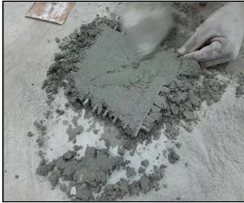
(iii) Pouring the mortar into the formwork
