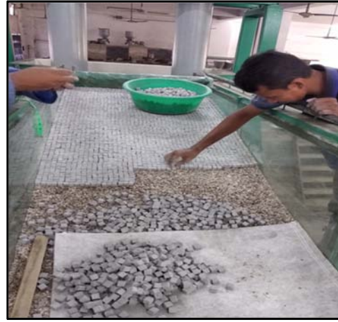
(vi) Placing of C.C. block
