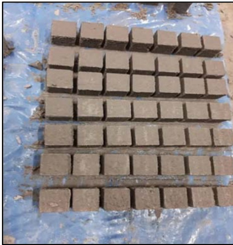
(v) C.C. block after removing the formwork
