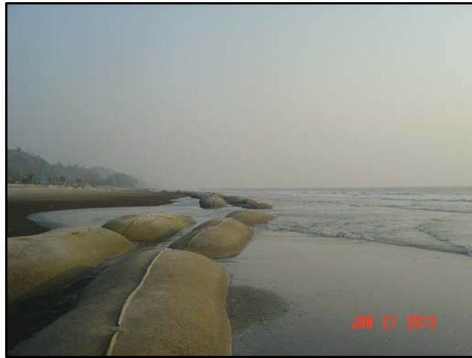
Figure 4.19: Emerged geo-tube settled in sandy beach (© M.A. Rahman)
