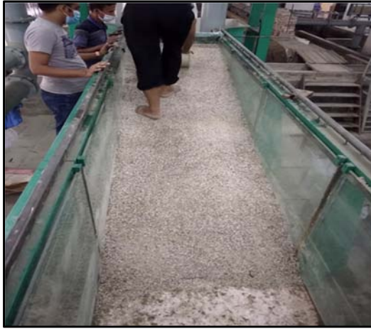
(v) Placing of stone chips
