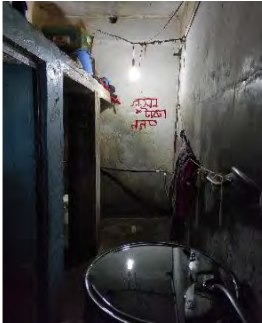
Photo B3: Water point-2 in the Tejgaon slum
