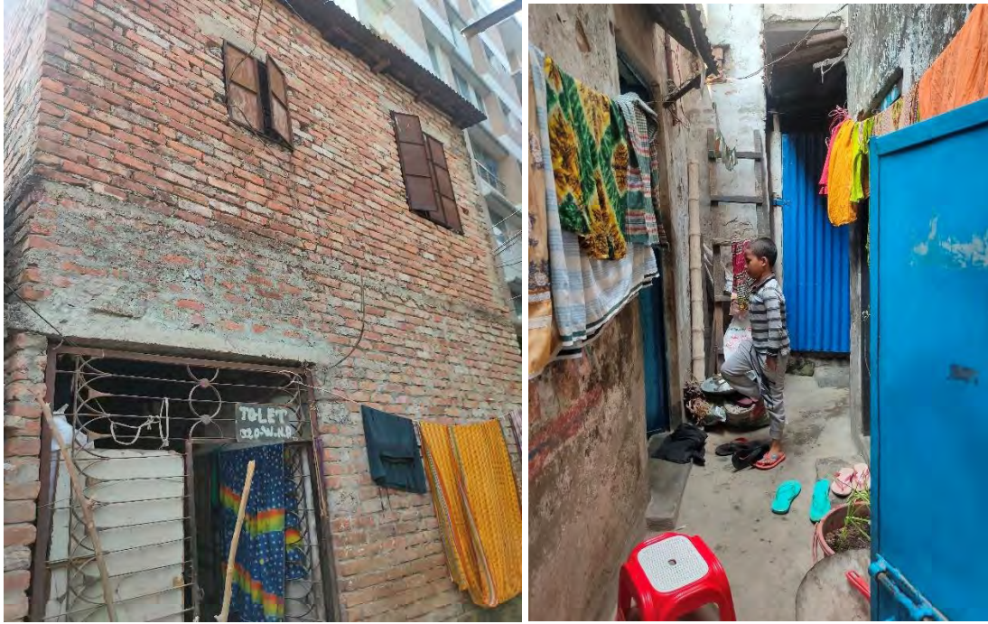
Photo B1: Sub-standard housing condition in the Tejgaon residential area
