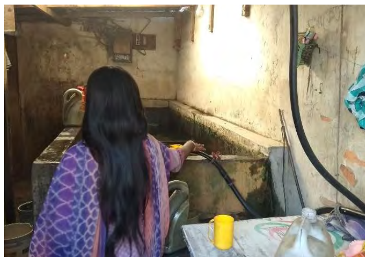
Photo B8: Water point-7 in the Tejgaon slum (closed at present)
