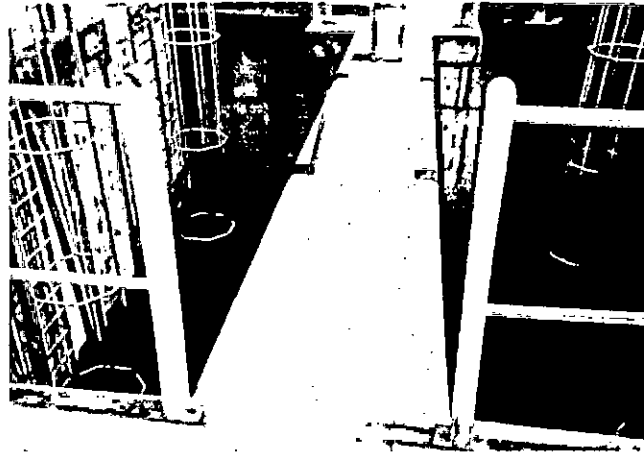
Photograph 4.1: Raw water intake pit at SWTP
