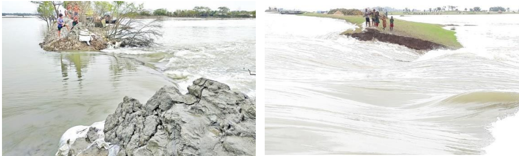
Figure 2-9: Breaching of embankments in the real world (source: google).
