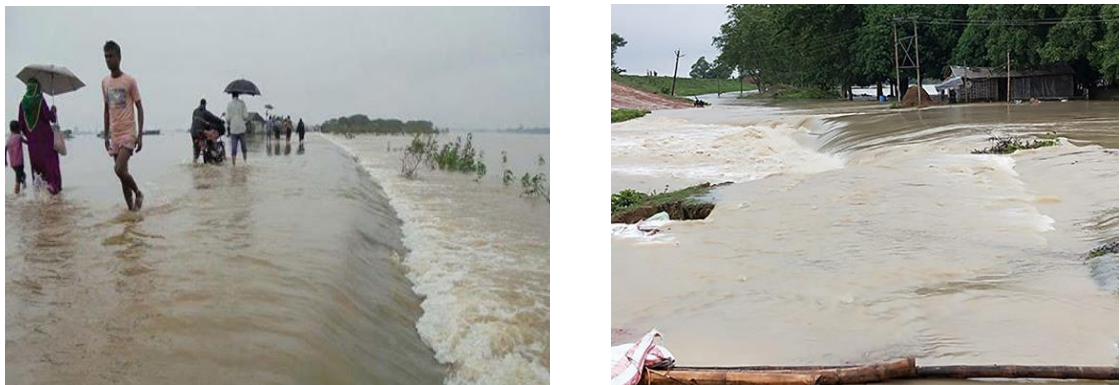
Figure 2-10: Flood water over tops embankment (source: google).
