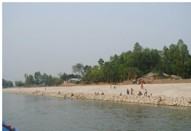
Figure 4-11: River Training works at Harirampur under FEREMIP project
