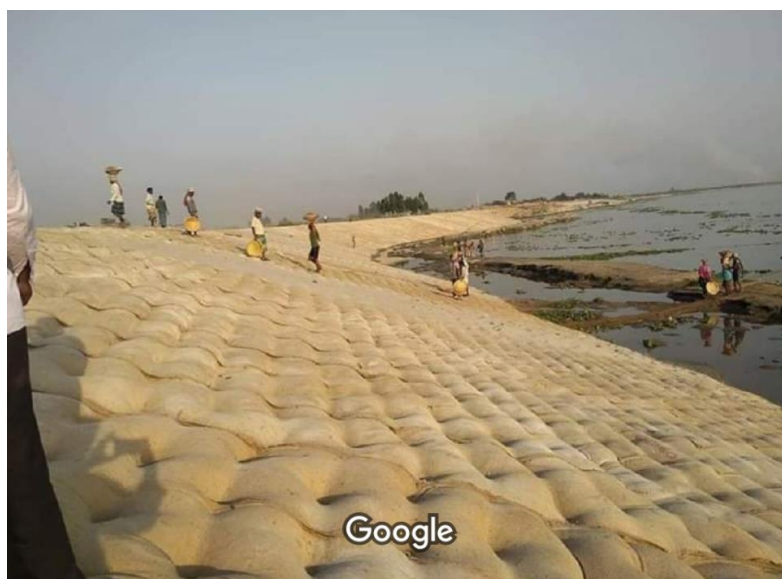
Figure 4-16: Flood Embankment Protection with Sand Fill Geo-Bag in FREMIP at Harirumpur (source: Google)
