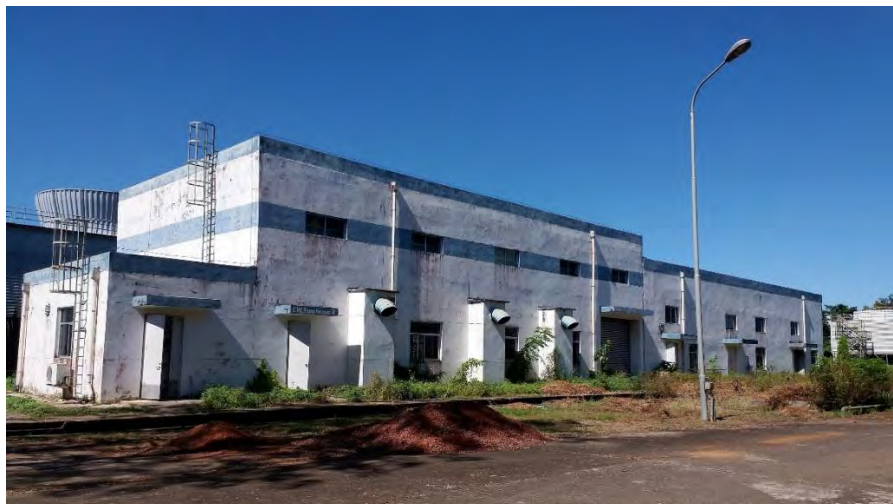
Figure 3.10: Closed cycle circulating water pump house.
