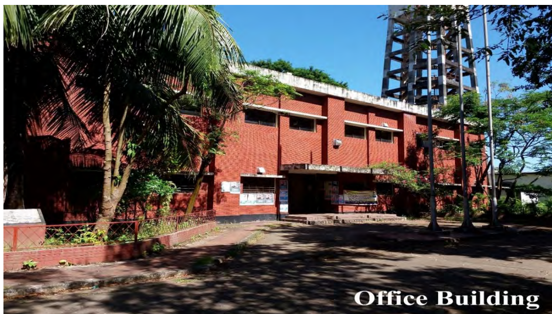
Figure 3.3: Administration building of the Fenchuganj Combined Cycle Power Plant.
