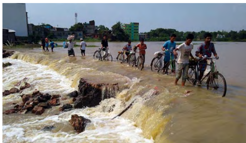
Figure 1.4: On rush of water from the hills in the Indian state of Tripura flooded a diversion road in Brahmanbaria's Bijohnagar upazila, disrupting vehicular movement on different regional roads (The Daily Star, 2019)
